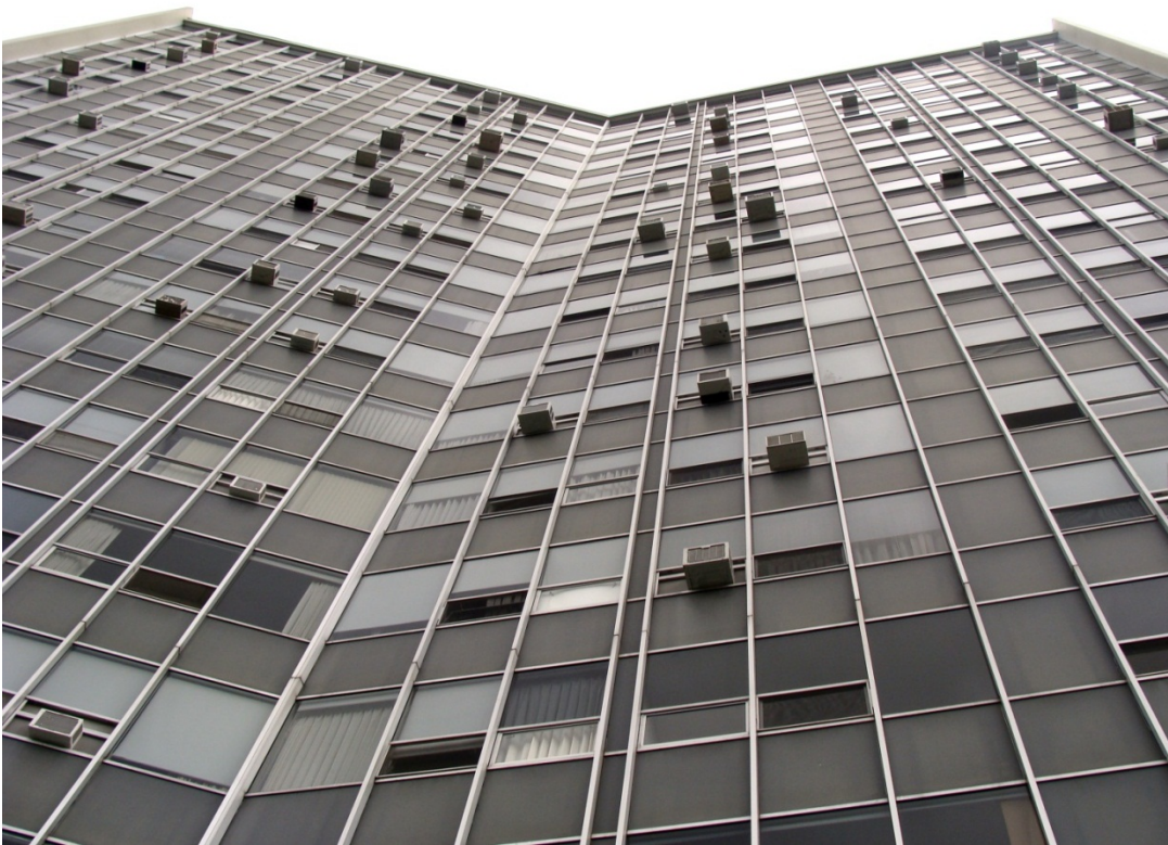
Figure 4.1. Southern façade of the Ya-Po-Ah Terrace, air conditioner units included.
