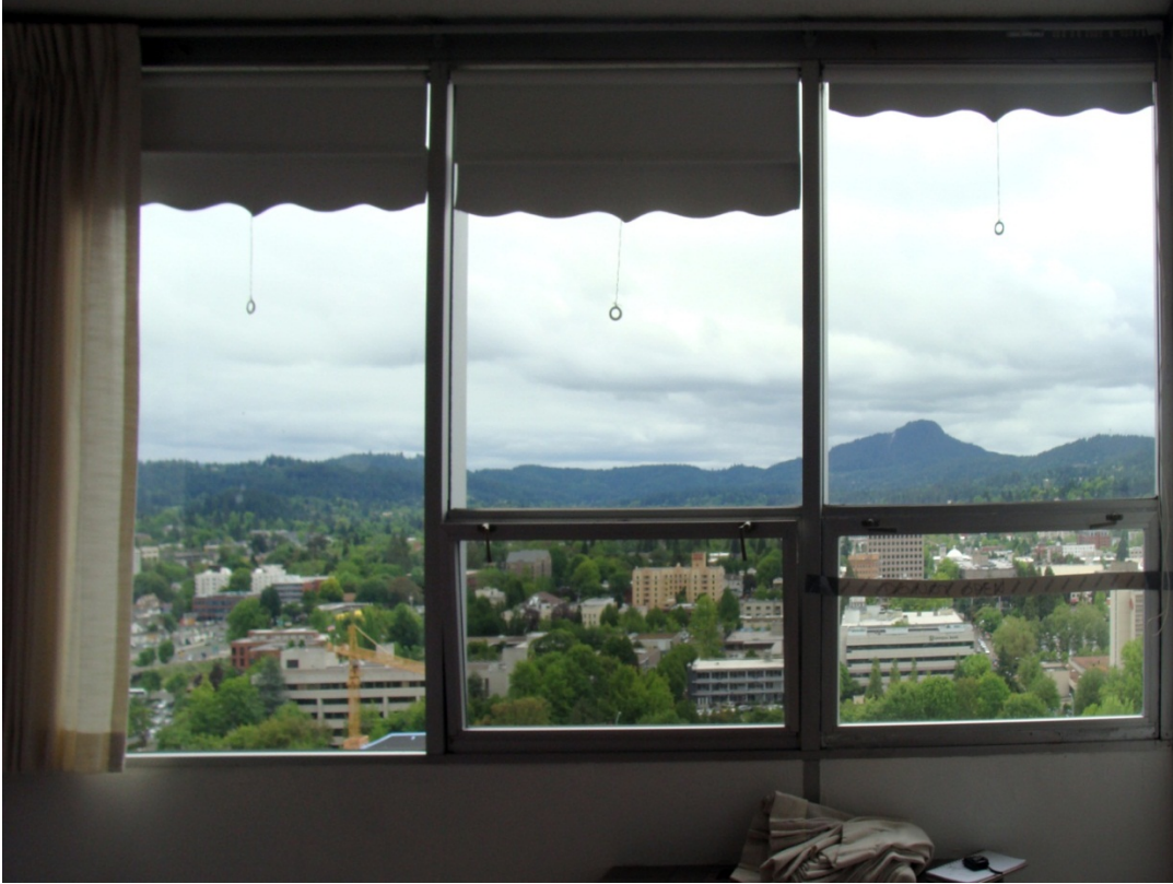
Figure 4.2. Interior view of the curtain wall system provided in each apartment of the Ya-Po-Ah Terrace.
