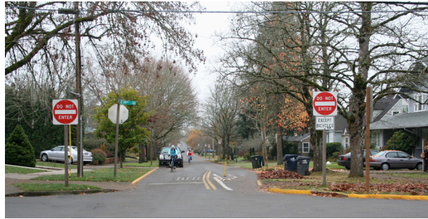
Figure 35: Pinch point at F Street intended to divert motorized traffic away from the entrance of the bike boulevard.
