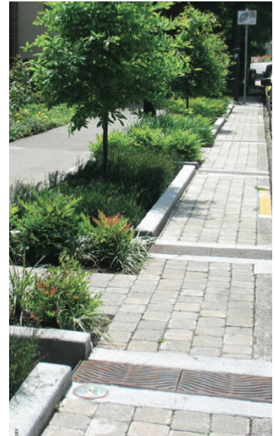
Figure 55: A storm water curb extension. Source: San Mateo County Sustainable Green Streets and Parking Lots Design Guidebook, 2010.
