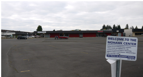
Figures 1-4: Current site conditions.
