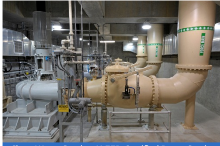
Clean Water Services' LEED Certified Pump Station
