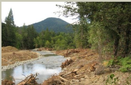
Post-Project: Downstream view immediately after channel construction
