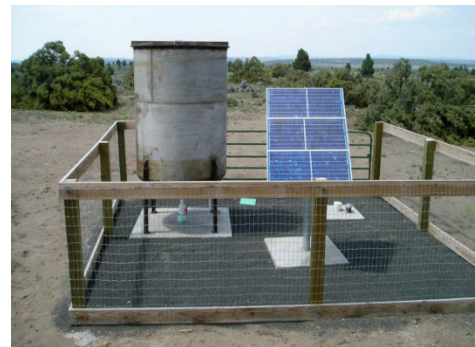
This off-grid solar livestock watering system provides a reliable source of water for livestock and wildlife, while also improving rangeland and streamside health.
