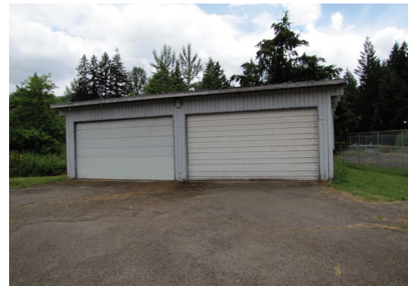
Figure 5.4. Accessory garage building
