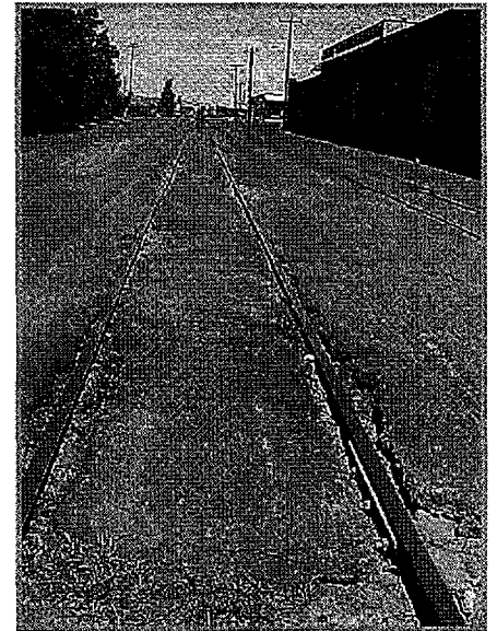
Deteriorating pavement on N. Bradford.
