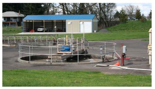
Figure 7-26: Silverton WWTP Primary Sludge Gravity Thickener
