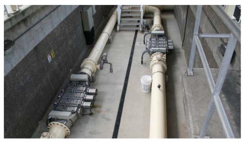
Figure 7-22: Silverton WWTP UV Disinfection System
