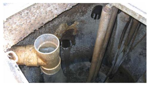
Figure 9-14: Manhole and Pump Station for Sidestream Recycle Flows
