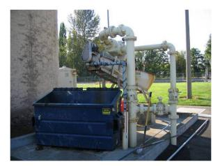
Figure 7-17: Primary Sludge Degritting Equipment
