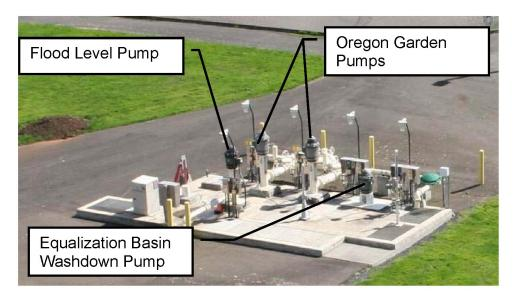
Figure 7-24: Effluent Pump Station at Silverton WWTP
