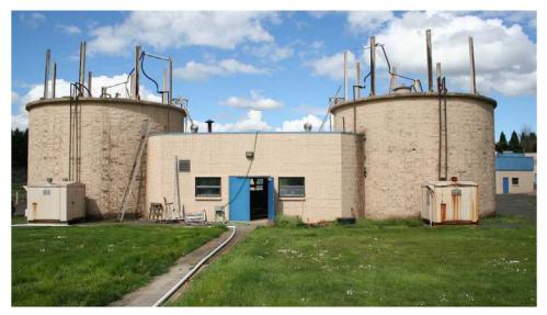
Figure 7-27: Silverton WWTP Anaerobic Digesters
