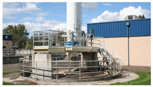
Figure 7-25: Silverton WWTP Dissolve Air Flotation Thickener
