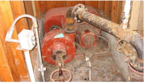
Figure 9-10: Primary Sludge Pump
