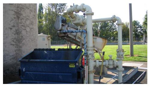
Figure 9-11: Silverton Primary Sludge Degritting Equipment
