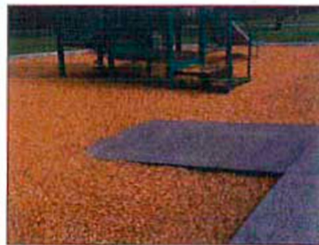
Figure 35. Example of ADA-compliant ramp into play area
