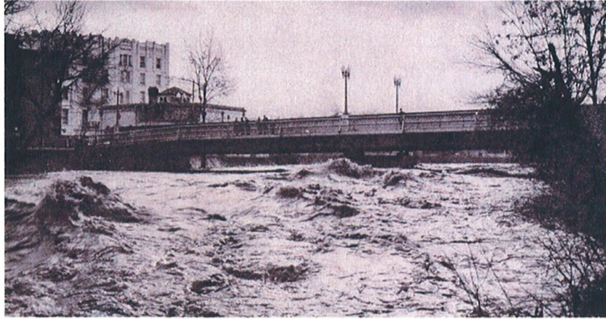
December 12, 1946 Right bank of Umatilla River, looking downstream at the Main Street Bridge. Flood discharge at 2:00 p.m., approximate peak flow of 13,700 cubic feet per second.
