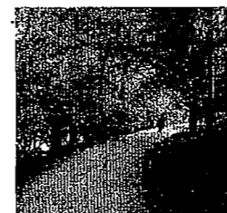
CRUSHED ROCK SECONDARY TRAILS PROVIDE A PERVIOUS, SOFTER SURFACE
