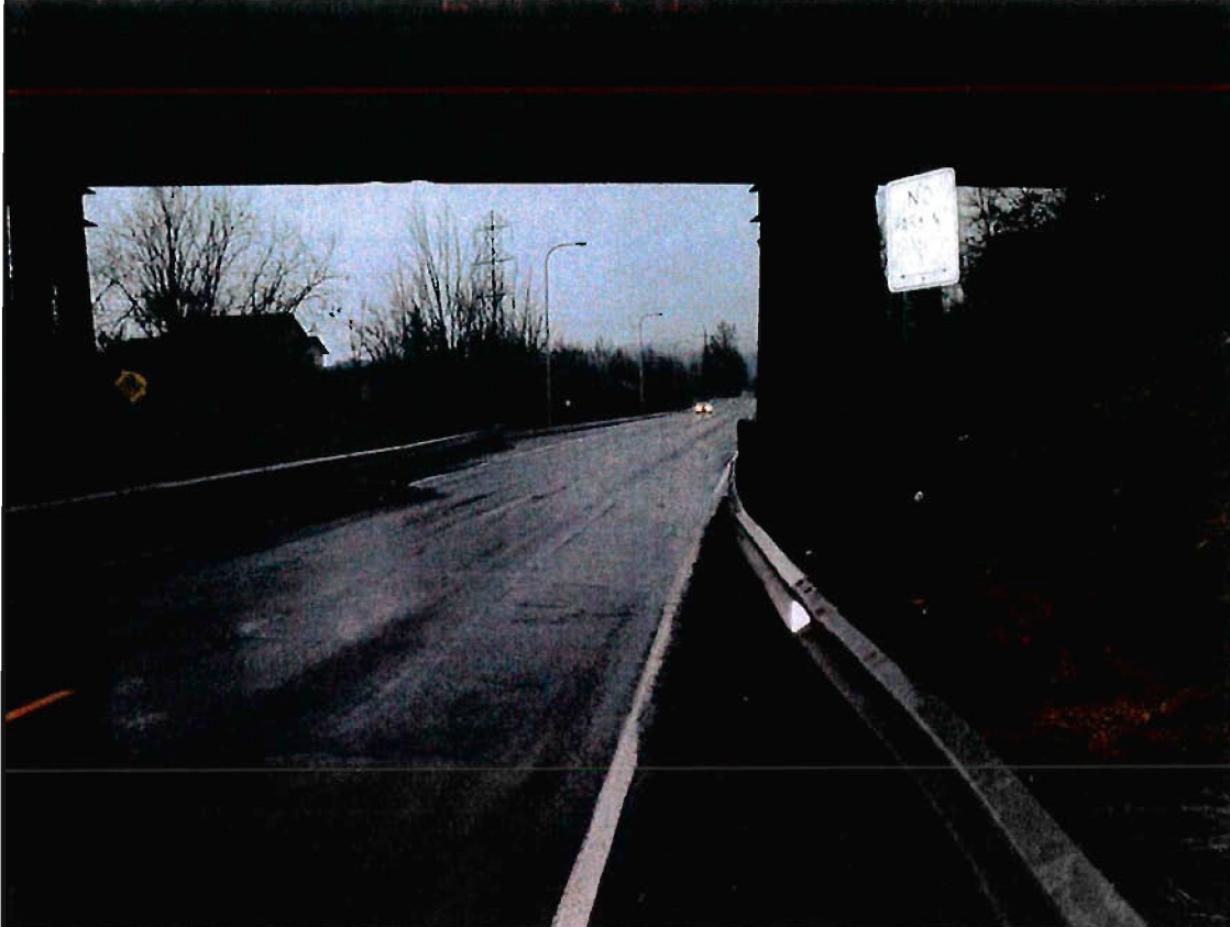
View - 223 rd Avenue Looking North, Railroad Bridge on 223 rd
