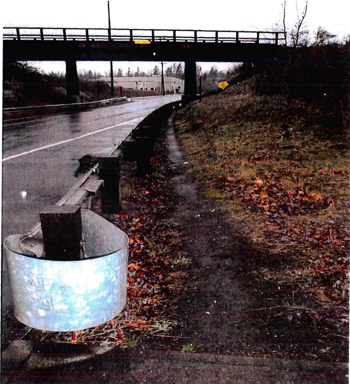
View - 223 rd Avenue Looking South at Railroad Bridge
