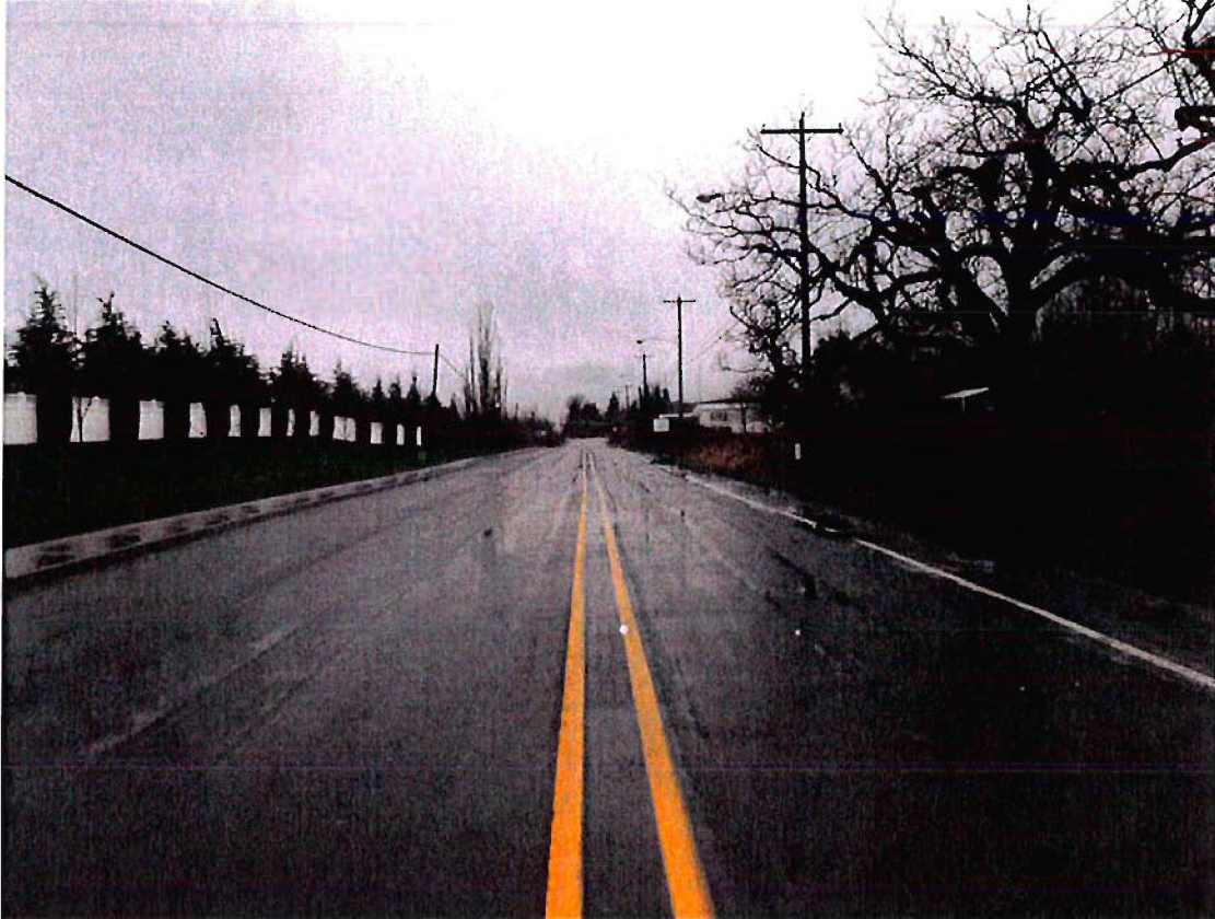
View - Sandy Boulevard Looking East, 1,000 Feet East of 223 rd Avenue
