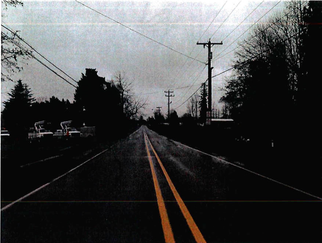
View - Sandy Boulevard, 850 Feet East of 223 rd Avenue, Looking East
