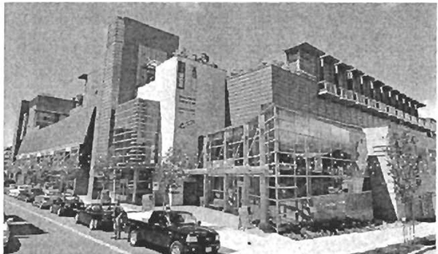
Fig. B.2.D.5: Weather protection is provided over the entry to protect customers from the elements.
