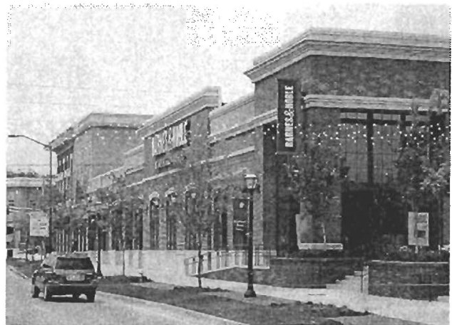
Fig. B.1.C.3.A: Design features create a vertical orientation in the facade.
