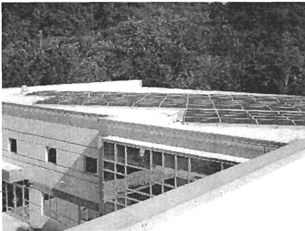
Fig. C.1.D.2: A roof using solar energy panels on a "white roof" to minimize heat gain and reduce cooling costs.
