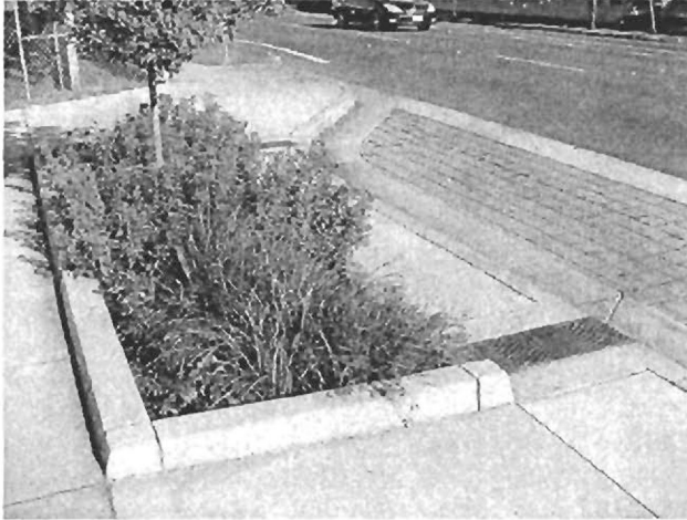
Fig. A.2.D.2.H.1: Amenity zone featuring a stormwater infiltration area and paved connections between parallel parking stalls and the sidewalk.
