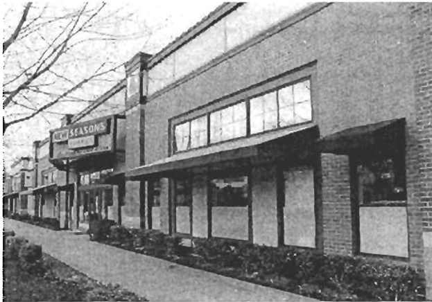
Fig. B.1.D.3.C: Slightly projected pilasters and recessed windows add surface relieve and shadow lines to the facade.
