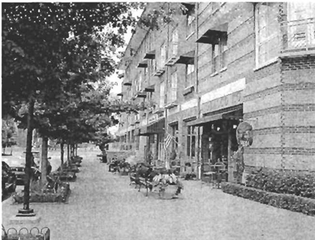
Fig. B.8.D.1(1): Multiple finishes of brick and stone are used together to establish texture in the facade.
