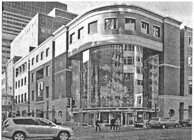
Fig. B.2.D.7: Increased levels of transparency at the building entry creates an attractive condition.
