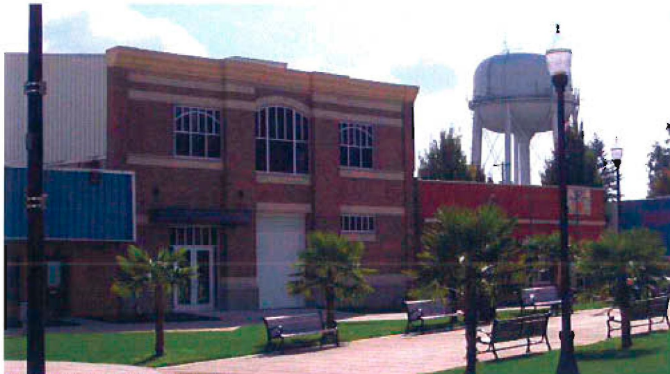
Priority Reuse of Association Building
