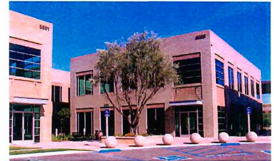
This office park development in California employs contemporary architecture and materials, however, the scale and facade patterning provides a human scaled and pedestrian friendly environment.
