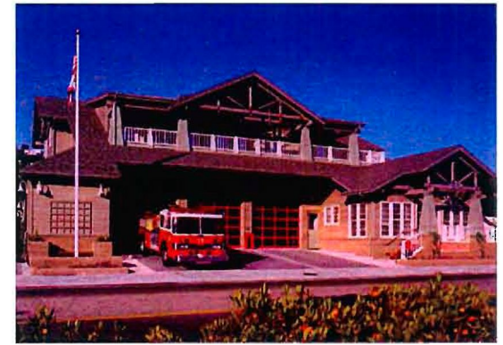
This Fire Station (Jackson, Wyoming) uses a dormer with a gabled detail and smaller front gables to achieve a varied roofline.
