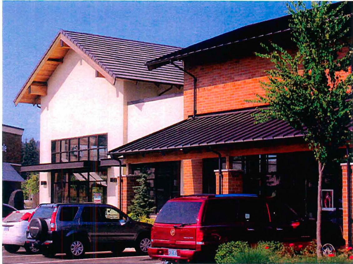
This local commercial development appears to consist of three buildings, which is achieved through distinct roof forms. The awnings and galleries add further detail that helps break up the massing.
