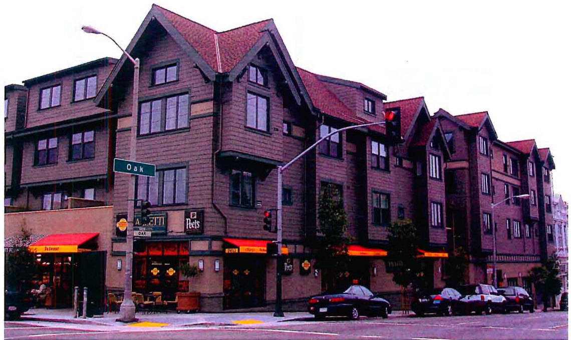
This large mixed-use development uses complex massing, varied rooflines, and proportions, detailing and materials to break down the scale of the building and evoke a residential character.
