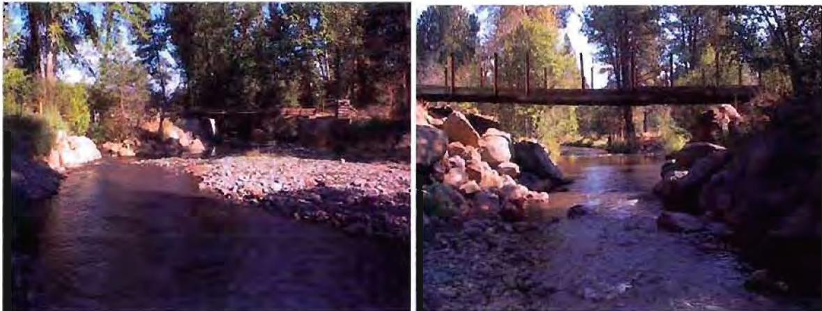
**Figure 15. Bridge in Segment 1A showing deposition upstream of constriction (left), and narrow bridge in Segment 3B (right) causing downstream scour and bank erosion.**
