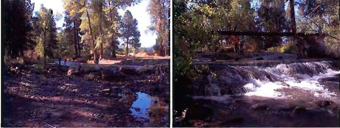
Figure 16. Boulder weir blocking side channel (left), and concrete weir (right) in primary channel, Segment 1C.
