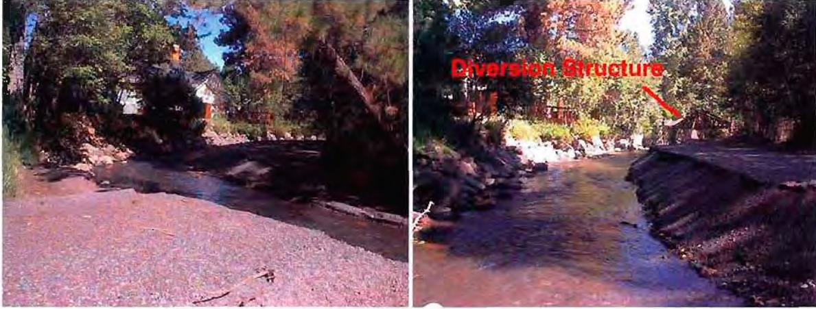
Figure 20. Sedimentation behind irrigation diversion located in Segment 1G.
