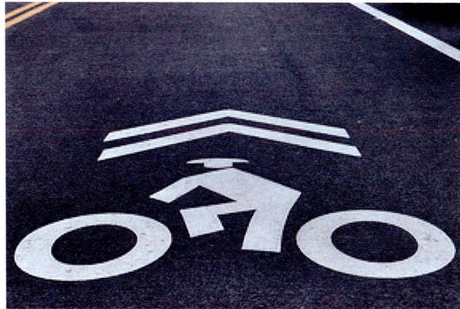
Example of a 'Sharrow' pavement symbol used to mark bike routes. Bicycles should travel over the 'sharrow' symbol. The placement, size and graphic design for sharrow marking can be found in current editions of the Manual for Uniform Traffic Control Devices (MUTCD). For neighborhood streets sharrows will typically be placed in the center of the travel lane.
