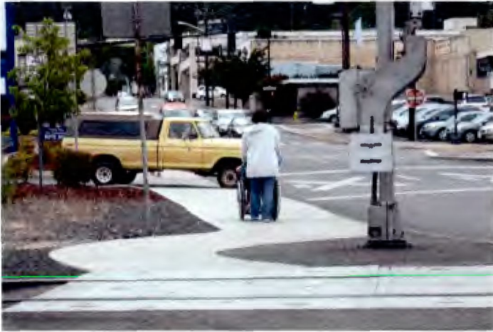
Appropriate design of railroad crossing locations can provide smooth transitions surfaces to reduce trip hazards. Railroad crossing locations can be improved with warning gates, lights, and bells to warn when trains are approaching.
