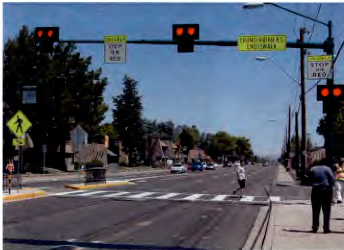
A H.A.W.K. signal is shown—High-intensity activated walk signal. These pedestrian activated street crossings couple signage, striping, and lighting to bring auto traffic to a stop so pedestrians can cross safely.
