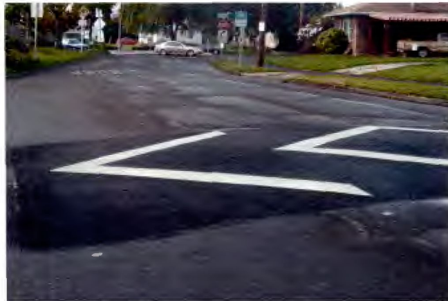
Speed humps are constructed to allow autos to pass over them safely and with minimal disruptions when traveling the appropriate speed limit. Speed humps are clearly marked to warn drivers and bicyclists of their presence.
