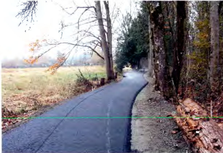
Paved trails accommodate a wide range of users and require less annual maintenance than unpaved trails. They are not preferred for equestrian trails.
