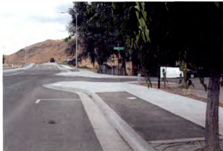
Curb ramps provide a smooth transition from the sidewalk to the street surface. Vibrotactile pads identify where pedestrians are to cross and provide a surface change identifier for visually impaired pedestrians.
