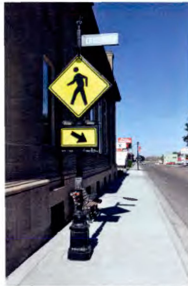
An example of a pedestrian-activated warning light. Flashing lights and highly visible signage warn drivers that a pedestrian is crossing the street.
