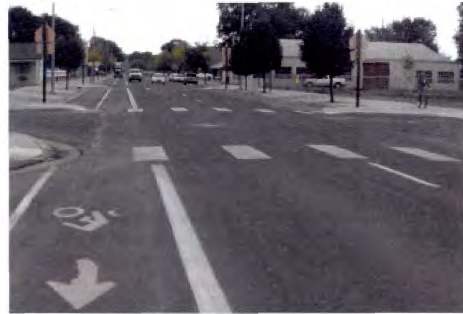
Bike lanes (shown here in Vale) provide increase visibility and safety for users. Standards and guidelines for the placement of signs and striping for bicycle facilities can be found in the Manual on Uniform Traffic Control Devices. Bike lanes should be at least 5 feet wide.
