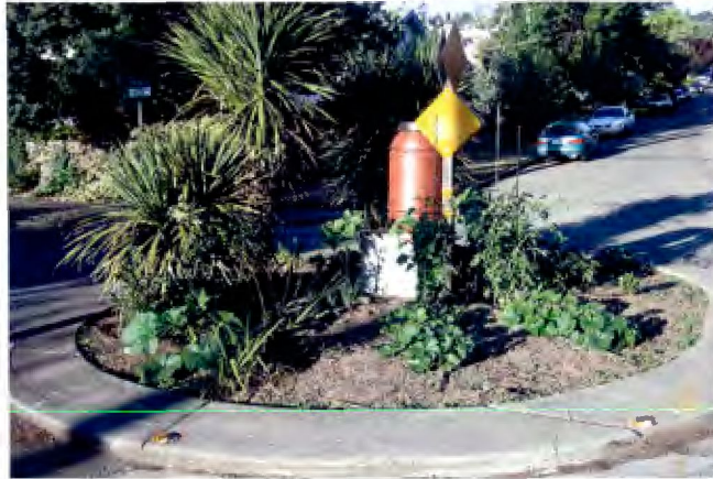
Traffic circles are placed in the center of intersections and provide a positive aesthetic value to neighborhood streets. Traffic circles also reduce the speed of autos and are constructed to permit emergency and maintenance vehicles access.
