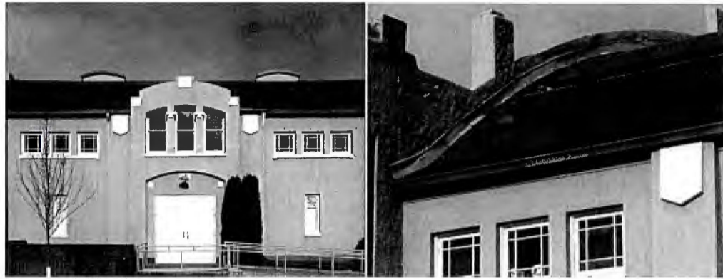
Historic Ashland Armory Solar Panels
