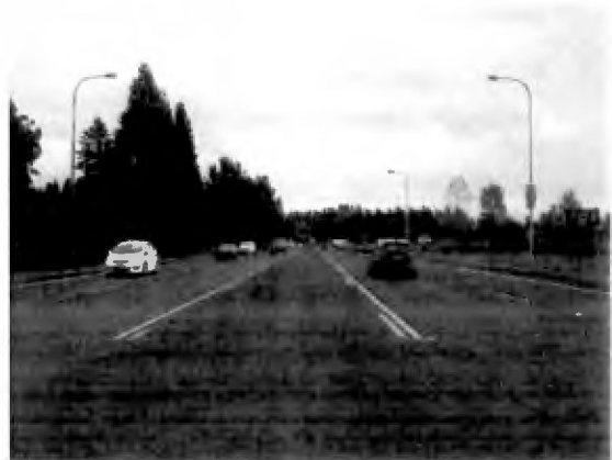
NE Glisan Street (Facing east)
