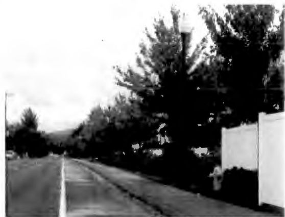
Improved Section of NE Arata Road (Facing east)
