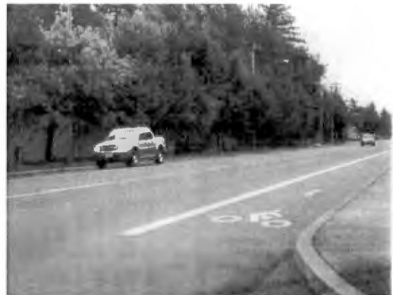
NE Halsey Street (Facing east)
