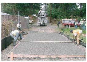
Porous concrete installation at NE 94th and Broadway. Additional porous concrete projects are planned to practice installation techniques, monitor their effectiveness and identify maintenance needs.
