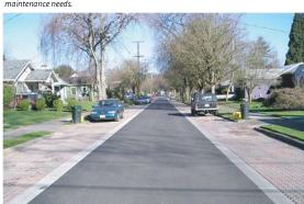
On SE 21st Avenue at Rex Street, permeable pavement allows water to go through the street surface and into the ground. It is the first use of this type of permeable paving material on a public street in Portland, although similar materials are used locally in parking lots and private driveways.
