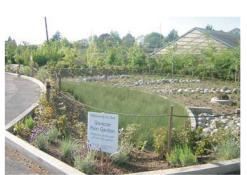
The Glencoe Elementary Rain Garden was built to address basement flooding and sewer backups from almost an acre of street and parking lot runoff.
