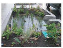
The New Seasons planters during a rain storm. Once vegetation becomes established, the design will remove about 1 million gallons of stormwater runoff from the combined sewer system each year.
