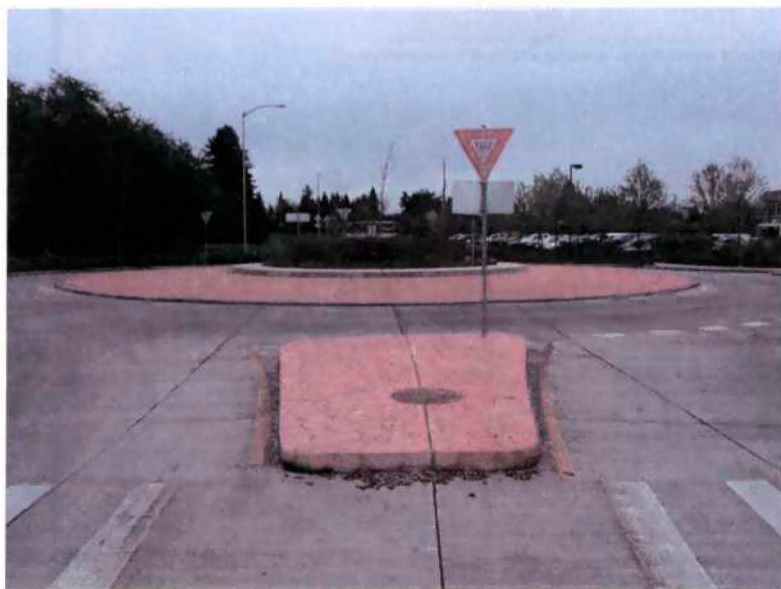
Figure 9B—The splitter island shown above has a textured concrete pattern but is not mountable. The proposed design includes mountable splitter islands.
