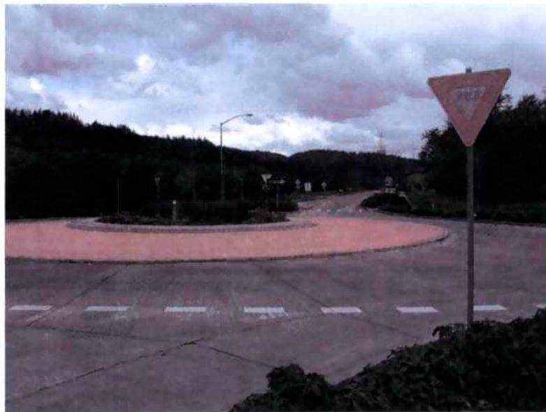
Figure 9A—The truck apron shown above has a textured concrete pattern and is mountable.
