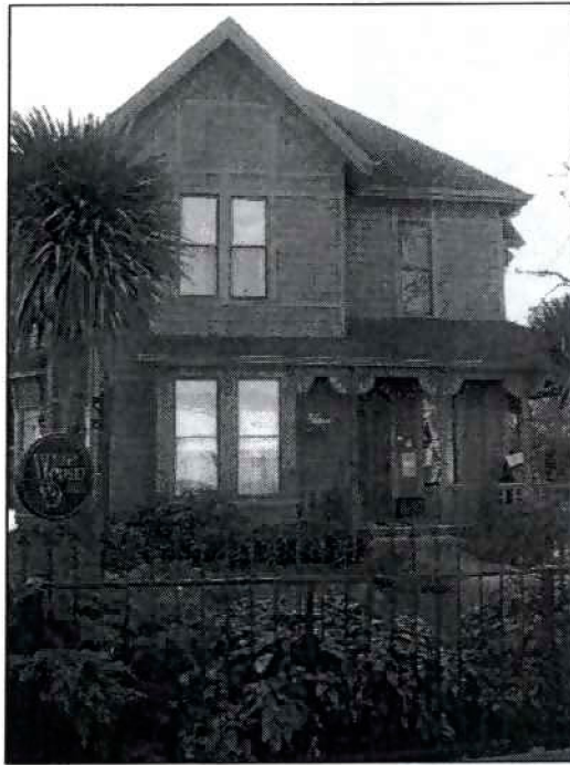
a. Figure 2.3.210.1.D.1 - Water Street Inn: 421 N Water St
