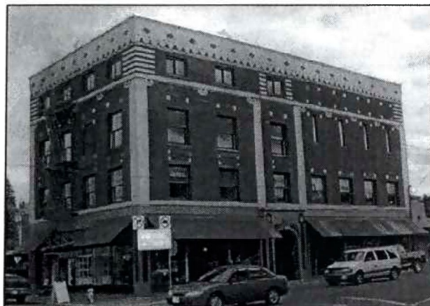
f. Figure 2.3.200.1.D.6 - Silverton Masonic Building: 101-110 S Water St
