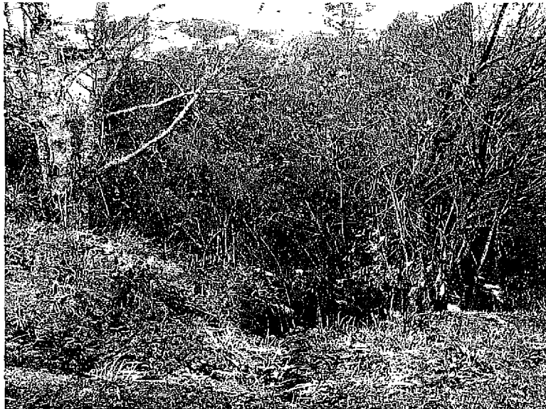
GROSS CREEK REACH 3: 9th STREET LOOKING NORTH
