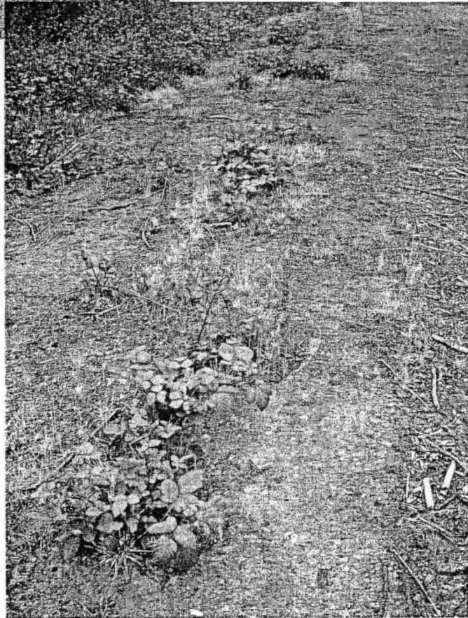
7 Asphalt road detail (apparently road constructed for heavy equipment before 1959)
