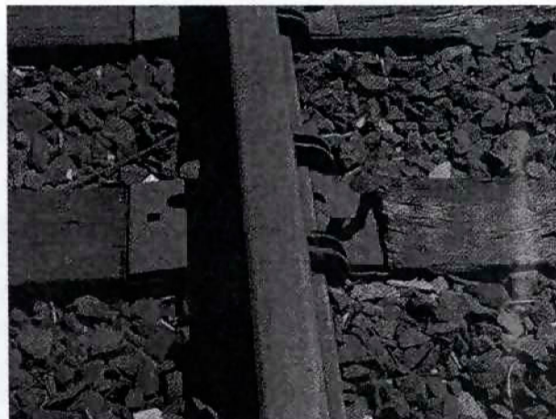
LOOSE RAILS AND SPIKES
