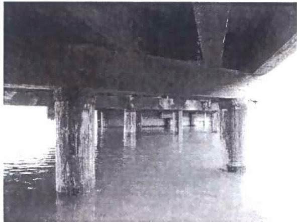
Millport Slough Bridge, view to north under bridge.
