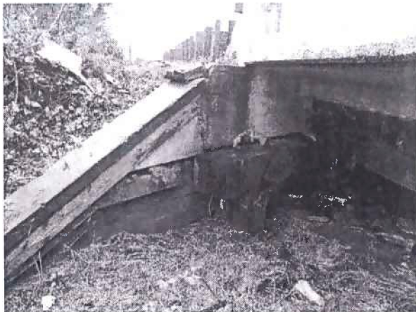
Southeast abutment, typical.
