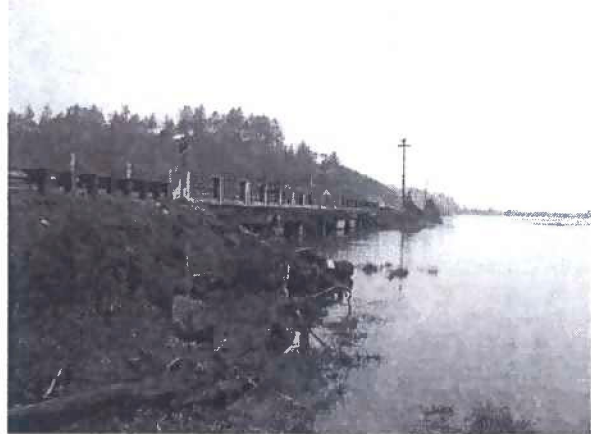
Millport Slough Bridge, view from northwest.
