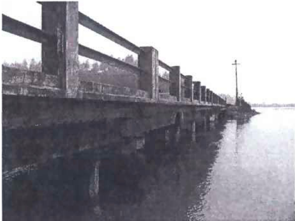
Millport Slough Bridge, view to south on west side.
