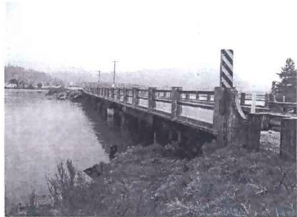
View to north on west side.
