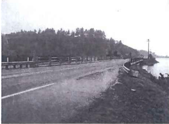
Millport Slough Bridge, view from northwest.
