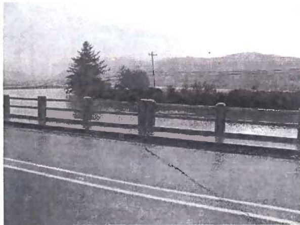
Typical bridge railing (altered).
