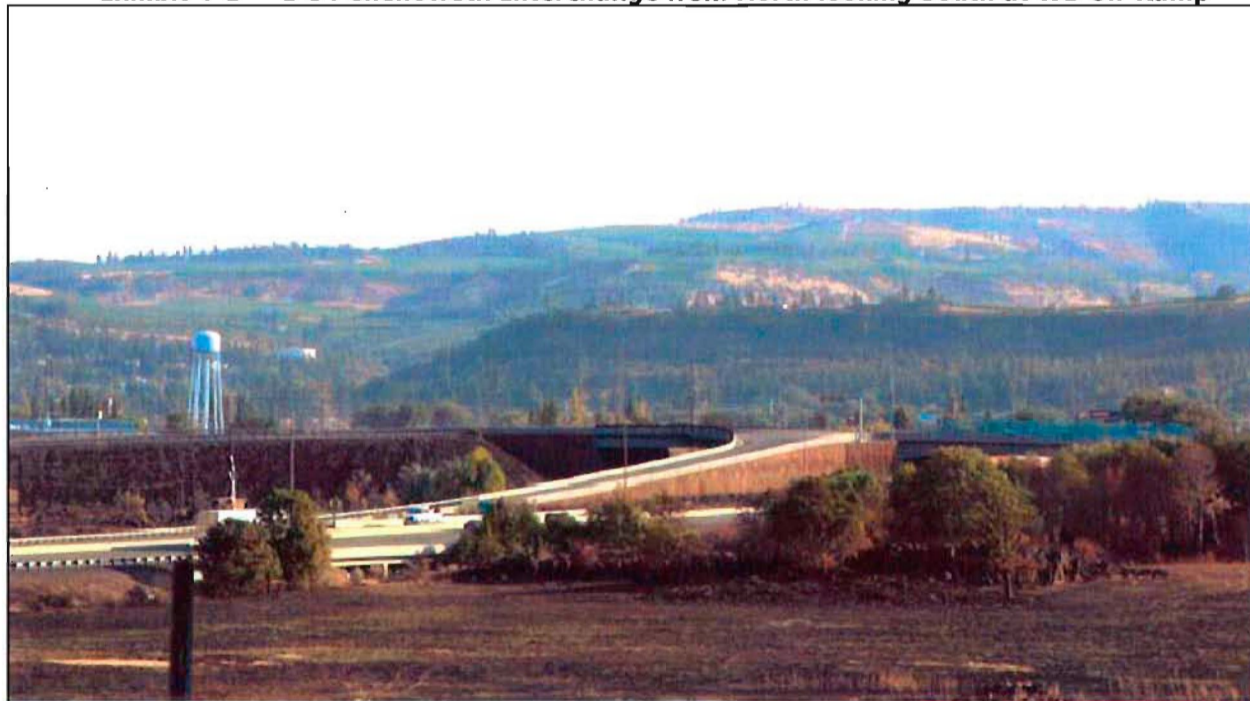
Exhibit 4-1 I-84 Chenoweth Interchange from North looking South at WB On-Ramp
