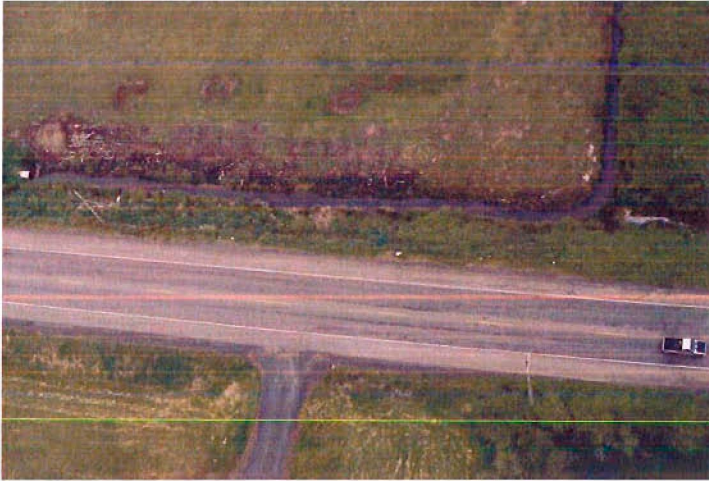
EXHIBIT 5 View of Current Drainage along the North-South Section of US 101 Business
