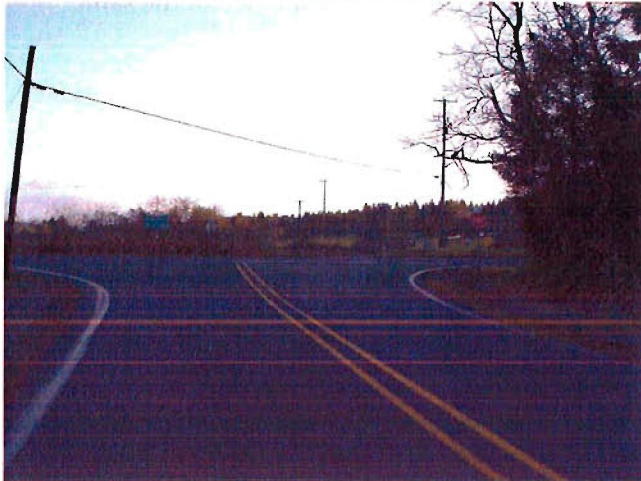
EXHIBIT 7 Airport Road at US 101 Business Looking South
