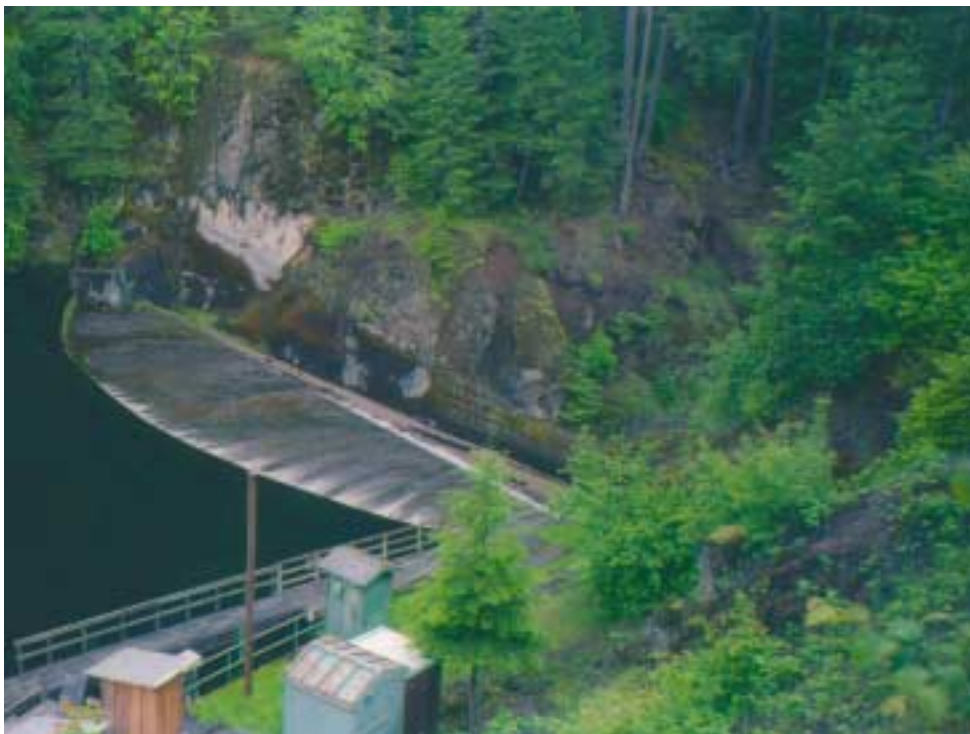
Figure 13. Dam at Lake Harriet on the Oak Grove Fork of the Clackamas above the mines. Photo by the author.
