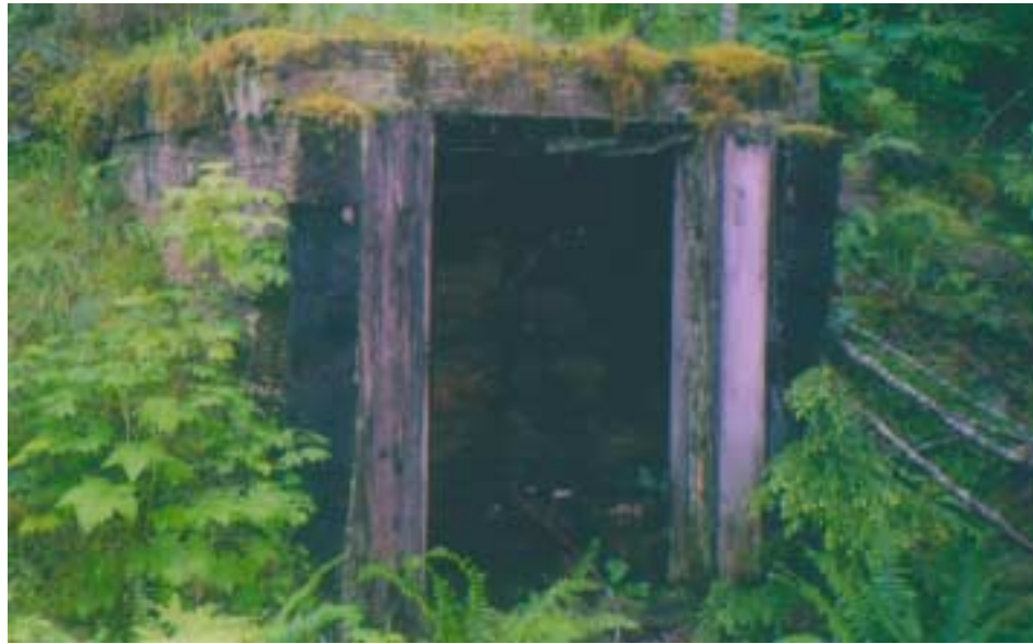
Fig. 7. Tunnel #3 at the Kiggins Mine. Photo by author.
