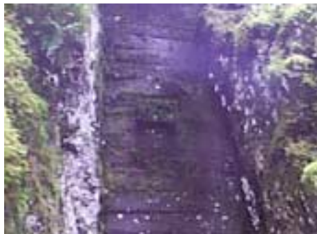
Fig. 14. Furnace at the Kiggins Mine. Note: The furnace has been built into a natural fissure in the area rock. Photo original by Bill Tompkins has been cropped by the author.
