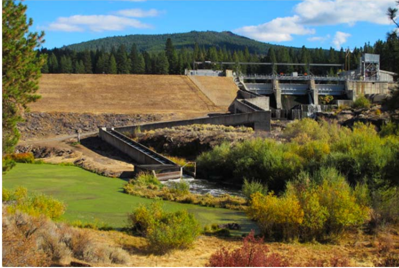
Figure 13. The John C. Boyle Dam, just downstream of Keno, Oregon.
