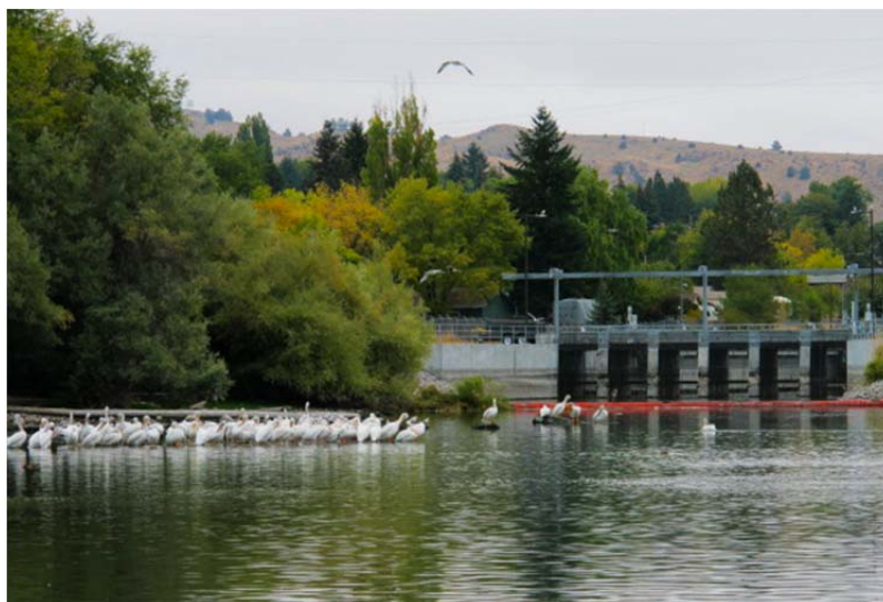
Figure 10. The A-Canal Headgates.
