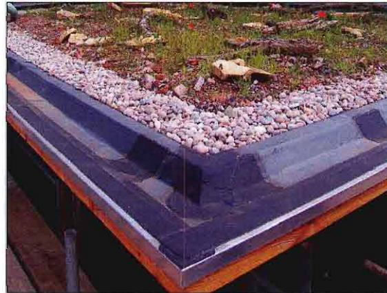
Appropriate - Landscaped Roof
