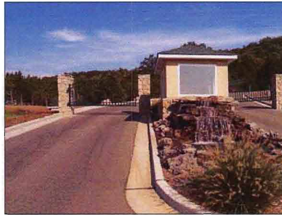
Inappropriate - gated and private streets
