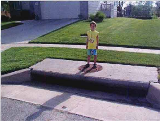
Inappropriate - Streets and Sidewalk drain to Stormwater Pipe
