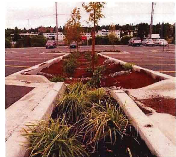
Swale Between Parking Stalls
