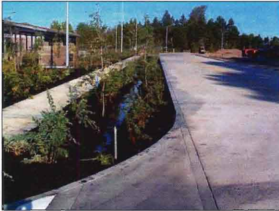
Appropriate - Surface Runoff Drains to a Vegetated Swale
