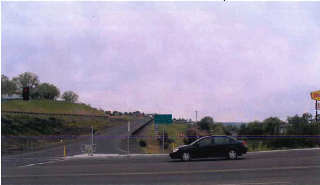
Exhibit 4-1 Eastbound I-84 On-Ramp from US 395
