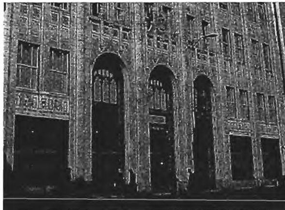
Fig 1.B.6.D.8.h: Higher bays, which extend two-stories in height, emphasise a highly-visible facade section.
