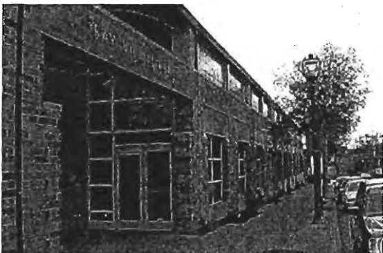
Fig. 2.B.2.C.3: Recessed windows create depth in the facade.
