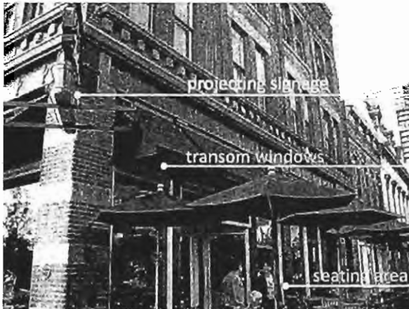
Fig 1.B.3.D.1: Transom windows, projecting signage and a seating area enhance the ground level of this facade.
