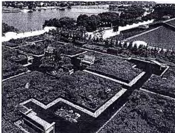
Fig 1.C.1.C.2: A modular vegetated roof system reduces stormwater and insulates the roof surface.
