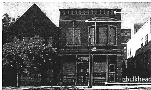
Fig 1.B.2.C.3: Horizontal elements, including a series of belt courses, the cornice and the bulkhead, establish rhythm in the storefront.
