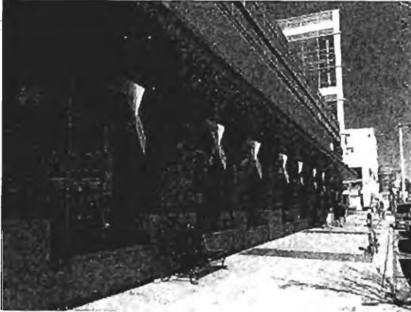
Fig. 2.B.3.D.2.c: Projecting sills and wall-mounted lighting fixtures add detail to this commercial building's facade.
