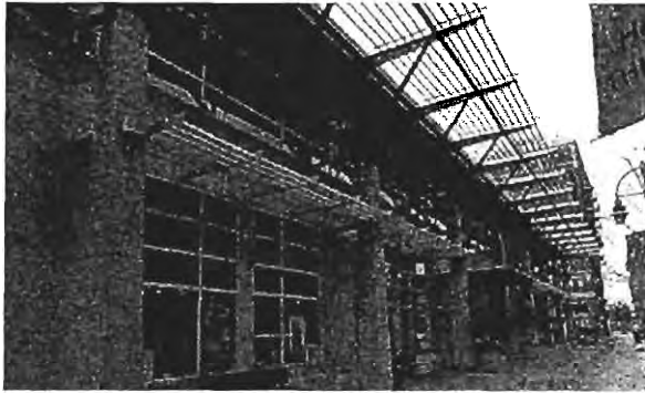
Fig 1.C.1.D.4.b.3: Solar shades are used to minimize summer heat gain while allowing passive heating in the winter.
