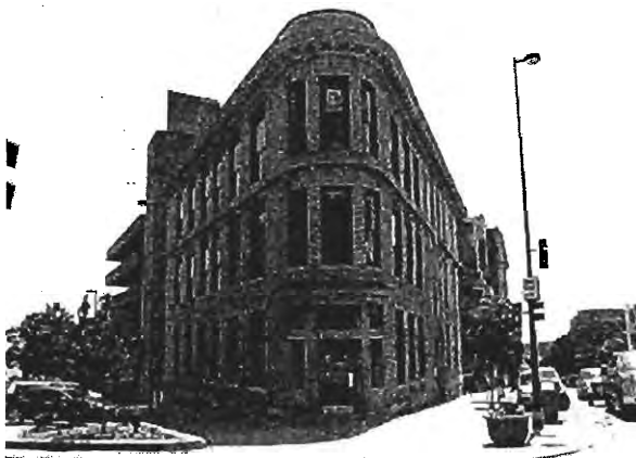
Fig 1.B.4.D.11: A renovated building in which windows were reinstalled.
