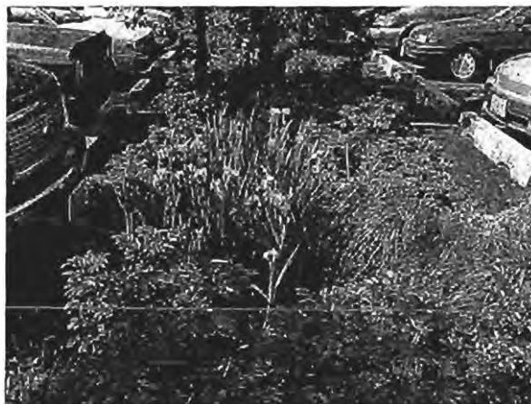
Fig. 2.C.1.C.1: A stormwater swale within a parking lot filters and manages the pavement run-off.
