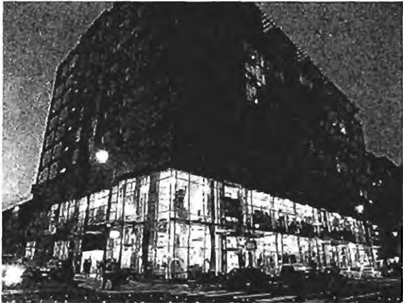
Fig. 1.A.10.D.1: Storefronts and exterior light fixtures create uniform illumination levels at the building entry.
