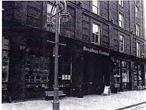
Fig 1.B.3.C.1: The ground level is enhanced by features including light fixtures, an awning over the door and transom windows.
