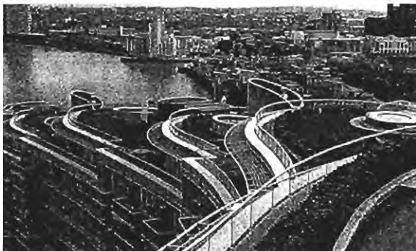
Fig 1.C.1.D.4.B: These green roof gardens help purify the urban air and lower urban air temperatures.
