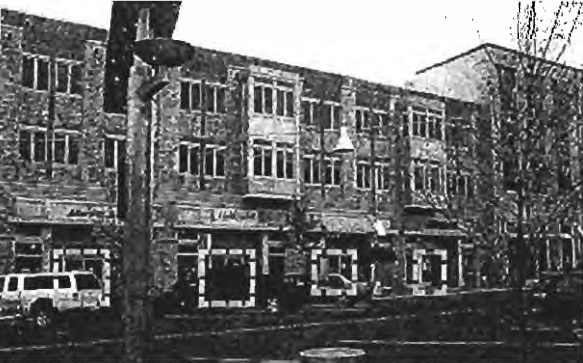
Fig. 1.A.4.D.4: A multi-tenant building over 120 feet in length with multiple street-facing entries.
