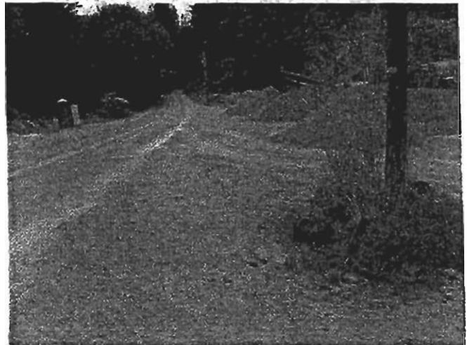
West end of road approach.
