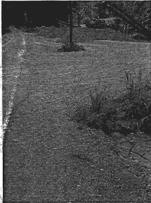
East end of road approach with culvert.
