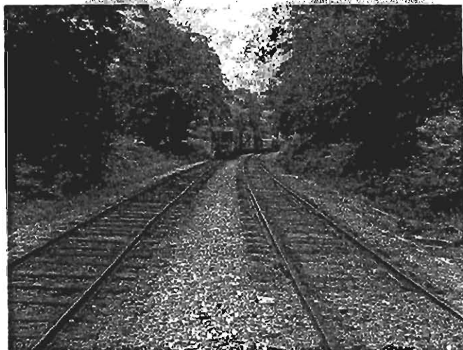
Port of Tillamook Bay Railroad track and siding.
