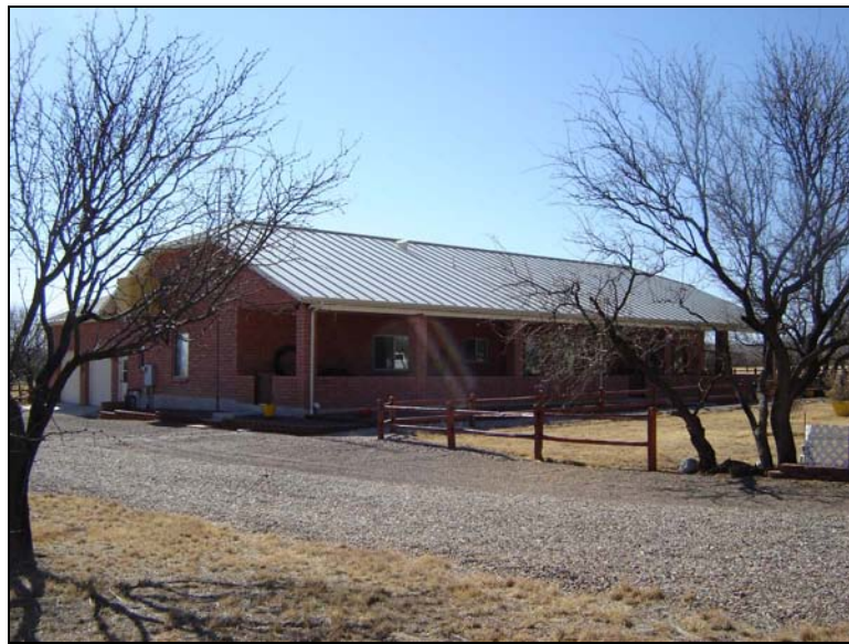
Photo 4.4 Firewise block construction, metal roof, and clearing around home
