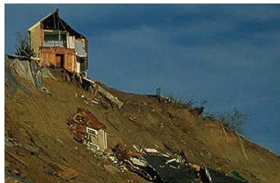
Landslides can damage or destroy roads, railroads, pipelines, electrical and telephone lines, mines, oil wells, buildings, canals, sewers, bridges, dams, seaports, airports, forests, parks, and farms.
