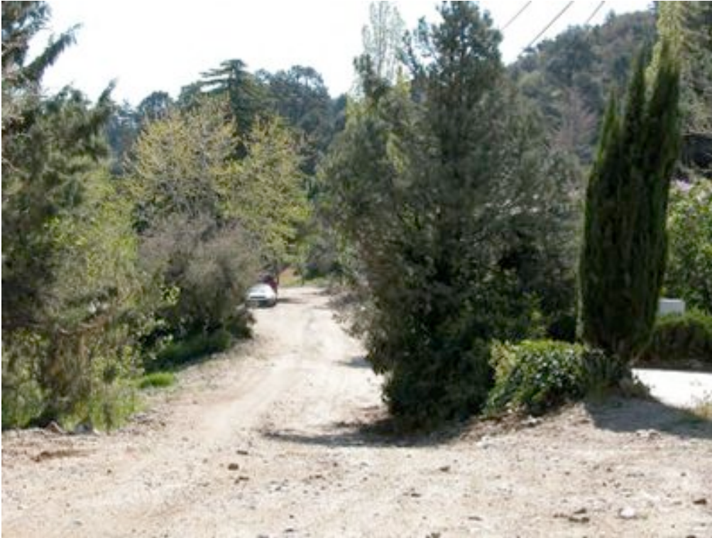
Figure 23: A typical “trail” found in Frazier Park which is a narrow unpaved road with several homes. This road is barely wide enough for a fire engine. Many of the trails are steeper and poorly maintained.
