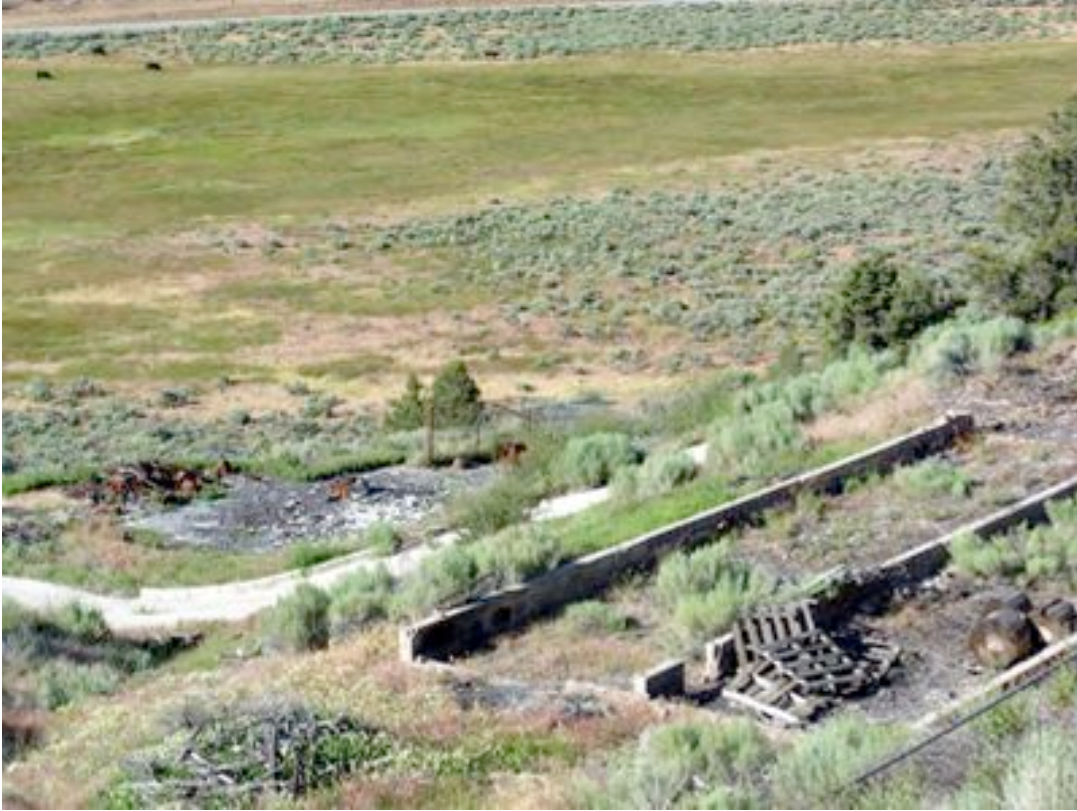
Figure 25: Burned debris and foundations are the only evidence of a wildland fire that destroyed three structures off of Whispering Pines Road on June 27, 1997.
