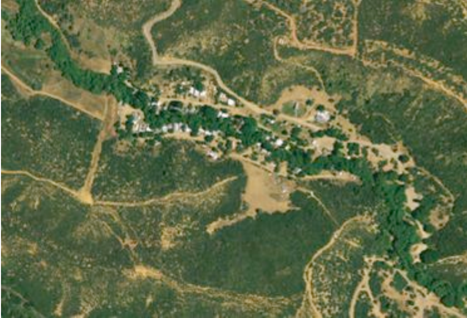
Figure 54: Looking down into Camp Scheideck indicates that the dwellings are located at the bottom of a bowl along Reyes Creek. There have been some attempts at reducing the threat of a wildfire as seen by the fuelbreak in the lower left of the community.
