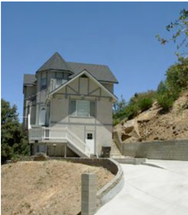
Figure 28: A new home in Frazier Park that utilizes many fire safe building materials. The roof is made of a Class A material that will resist ignition. The eaves are boxed in and the windows appeared to be multi-paned. The home is built with stucco that could stand direct flame impingement. Although the vegetation in the yard to the right appears to have been modified, the tree in the left could compromise the home due to the open construction of the stairway.
