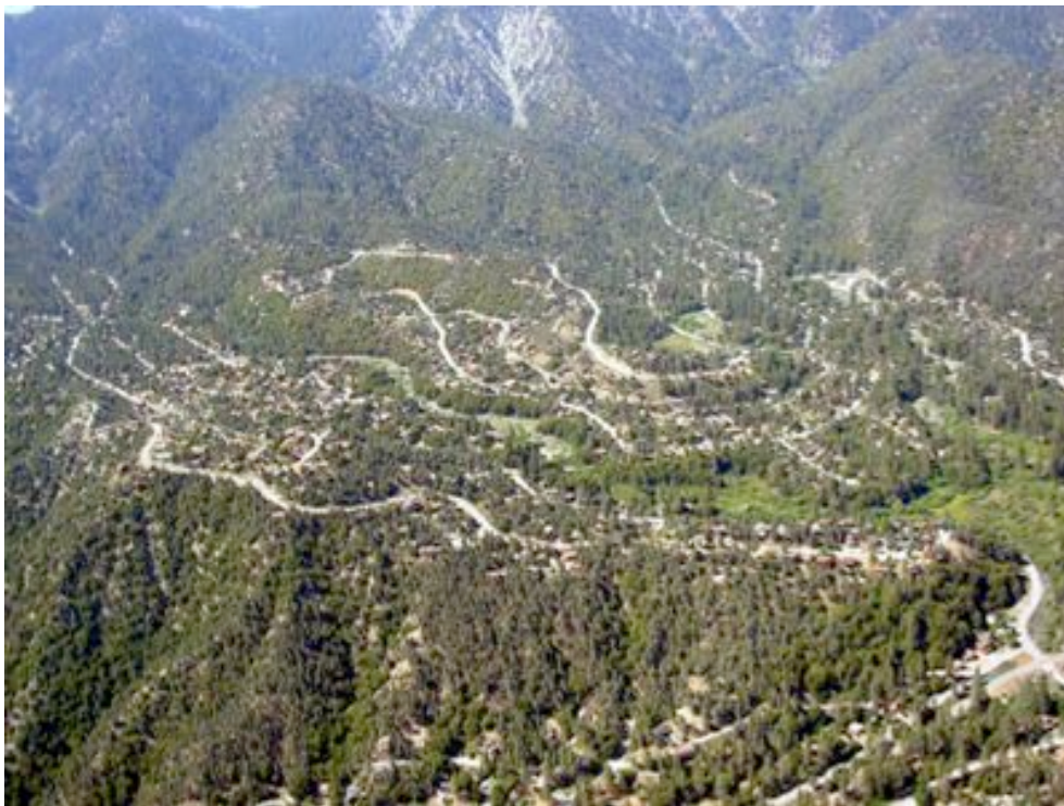
Figure 46: The challenges of protecting Pine Mt. Club from a wildland fire become obvious in the photo. Heavy fuel types, steep terrain, and several dwellings with limited access combine to create a community at risk.
