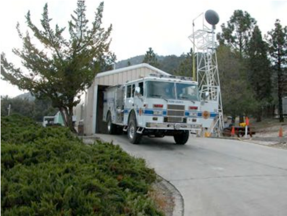
Figure 32: The area covered in juniper left of the driveway at Fire Station 57 would be an excellent place for a fire safe garden.
