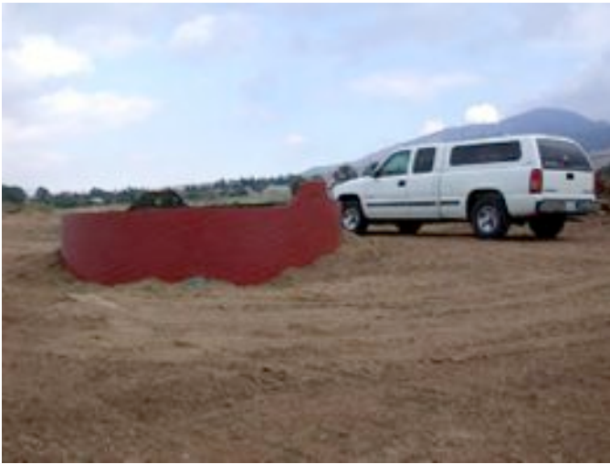
Figure 56. The metal dip tank that is partially underground used to fill helicopters during a wildland fire. The tank is pumped with a valve attached to a water main for fast filling.
