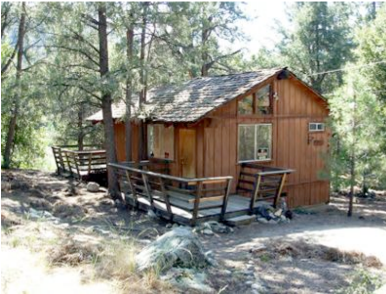
Figure 27: This dwelling in Pine Mountain Club not only has a wood roof but it is covered with pine needles making it very susceptible to a wildland ignition.
