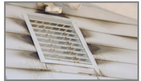
Vents are vulnerable openings that must be protected in order to harden your home. This is a great retrofit opportunity.
