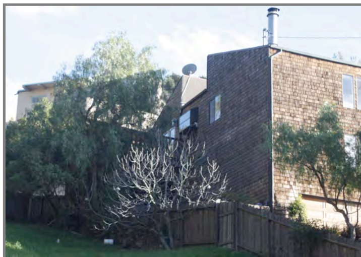
Urban fuels (flammable and dead vegetation, and a wooden fence) against wood-shingle siding, a dangerous combination.
