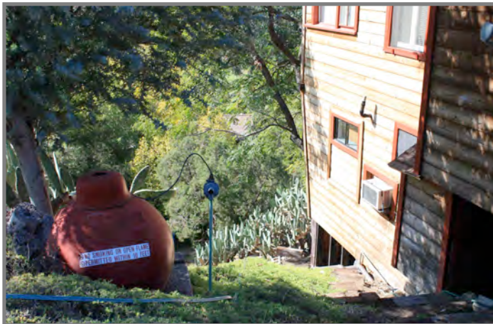
These fuels are too close to this wood-sided house. The open areas under the home should be sealed off.
