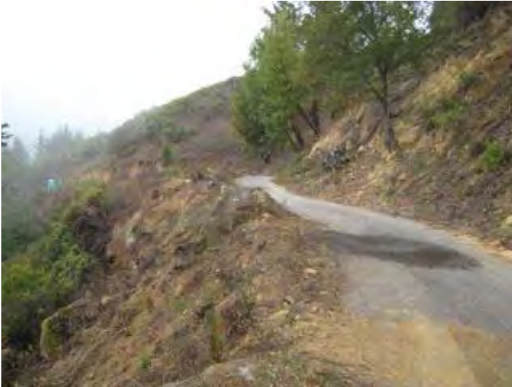
Fuel break on midslope road in Las Cumbres, Santa Cruz County
