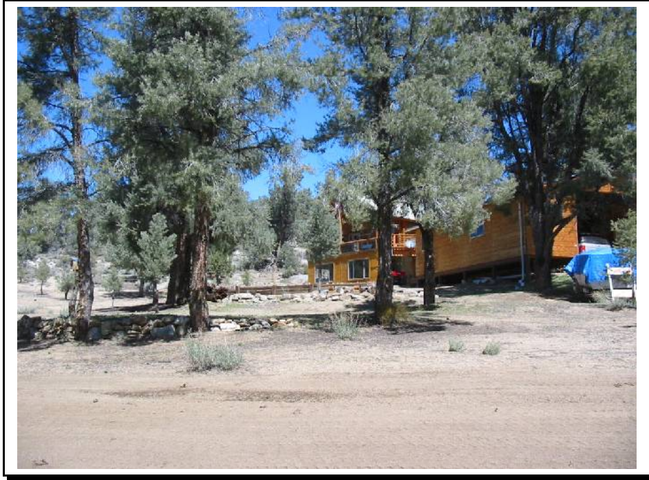
Log home with good clearance, space under shed should be sheeted.
