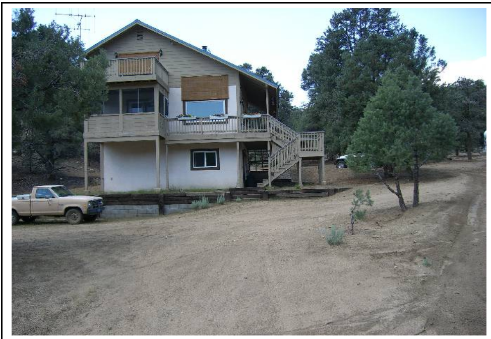
Structure pictured has good clearance, non-flammable siding, metal roof, composite deck, and emergency water supply with hydrant.
