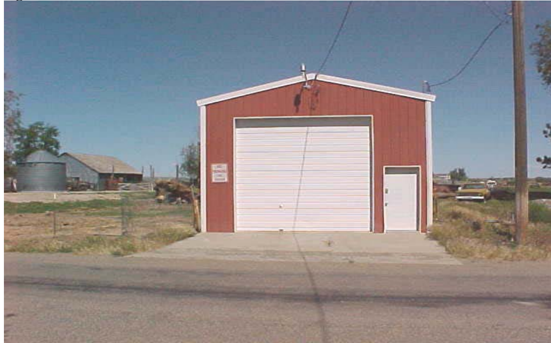
Figure 14: Shoshone Fire Station #2
