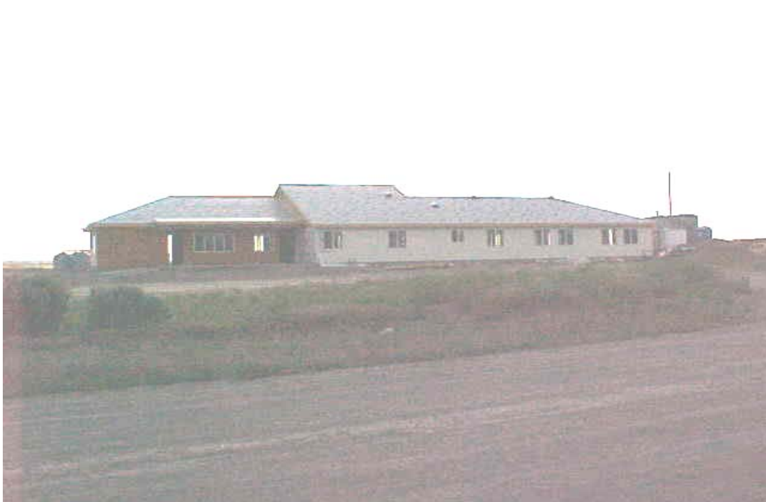
Figure 19: New Kimama BLM Station (Under Construction)
