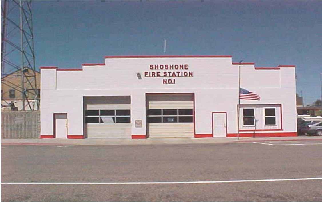
Figure 13: Shoshone Fire Station #1
