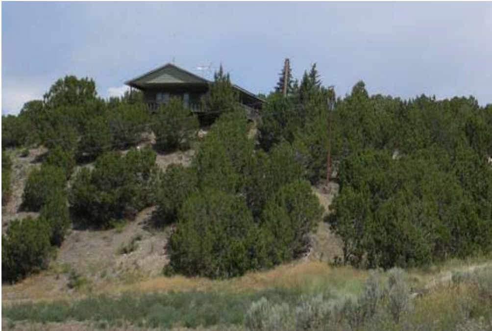
Figure 7. Juniper Addition showing fine fuels, heavy juniper and no survivable space.
