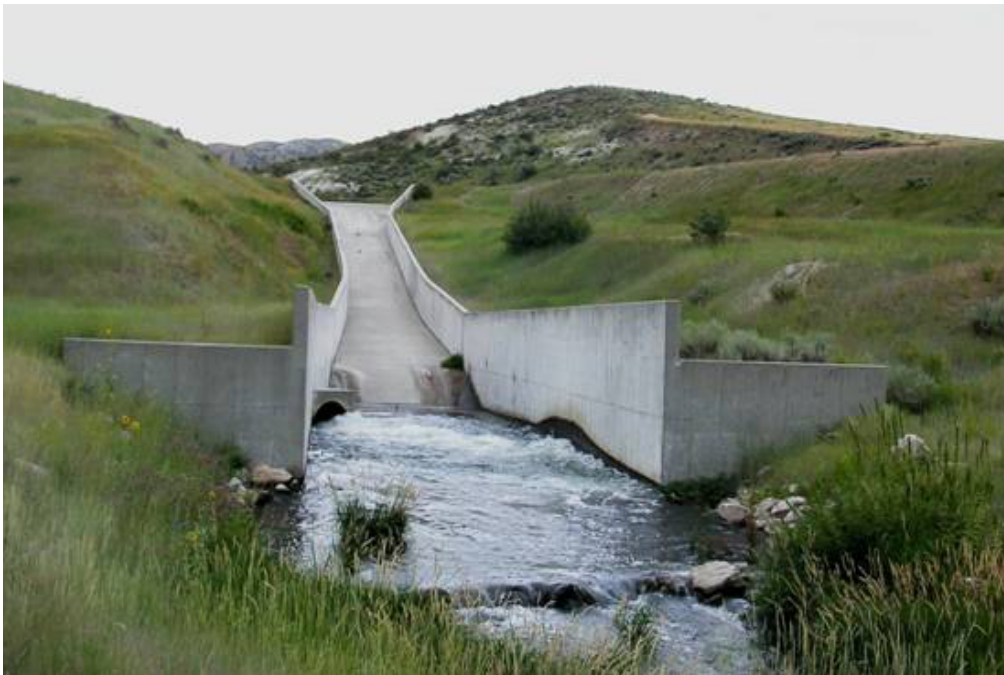
Figure 12. Devil Creek Reservoir outlet showing dry hydrant or drafting location.
