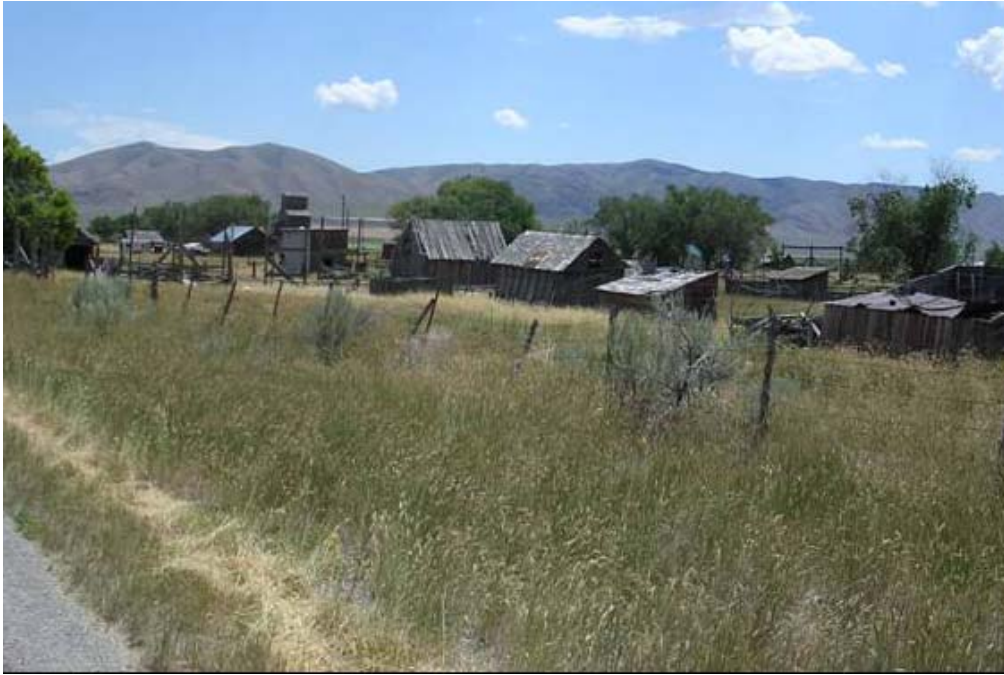
Figure 9. Abandoned structures within Holbrook showing fine fuel buildup and low survivable space.
