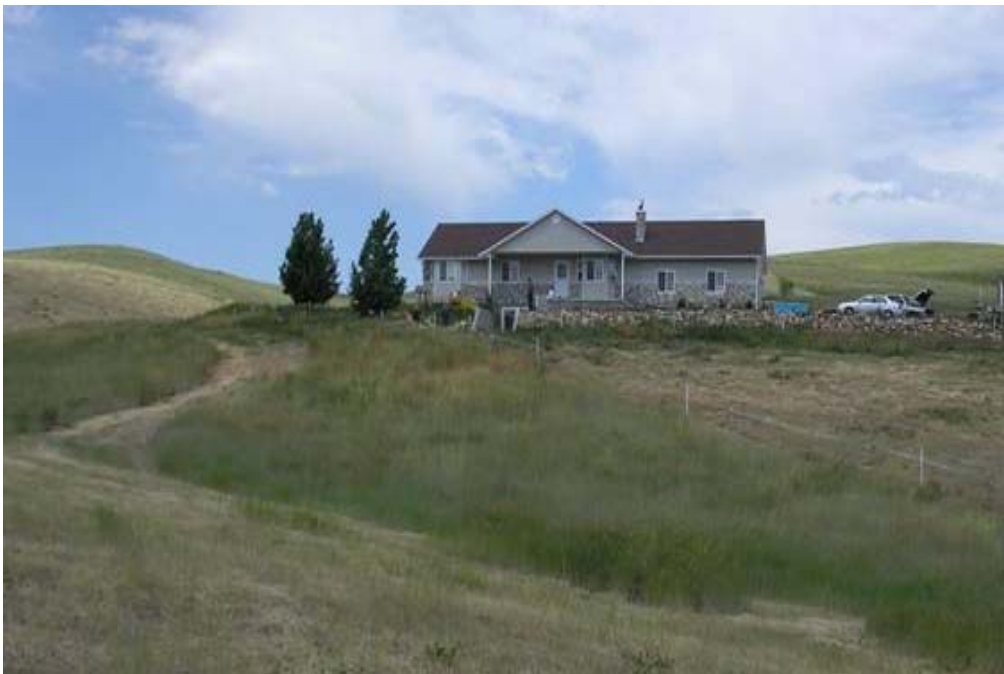
Figure 6. New Canyon Subdivision home showing fine fuels and moderate survivable space.
