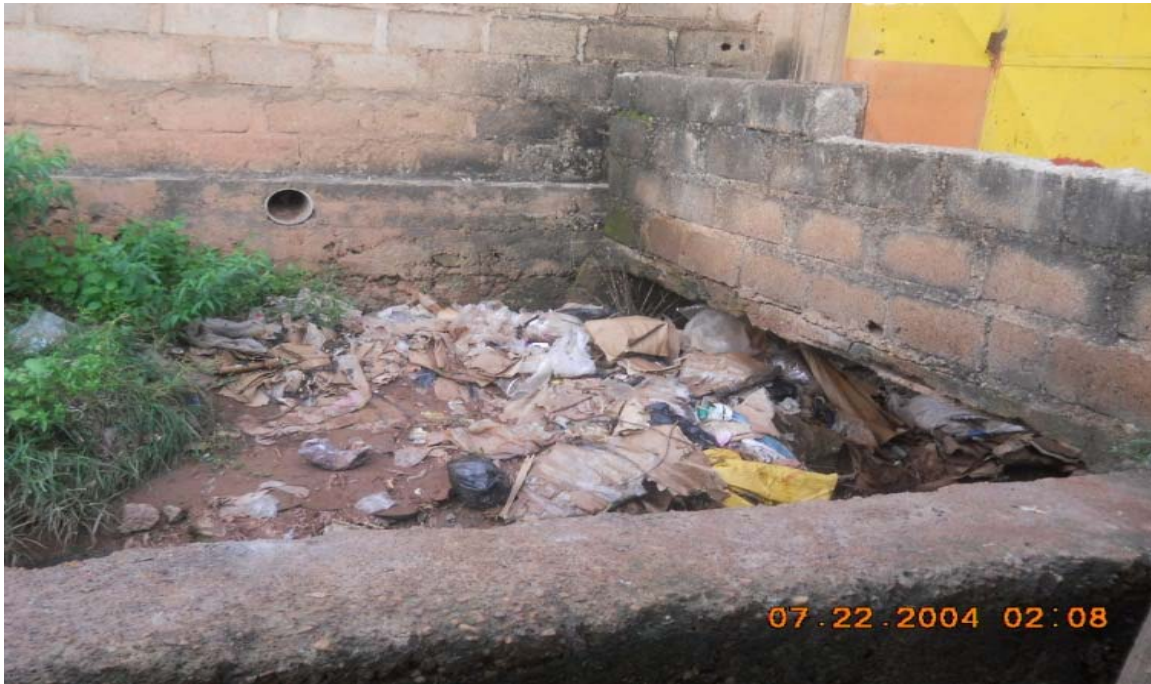
Drainage Blocked by Plastic Waste in Bougouni
