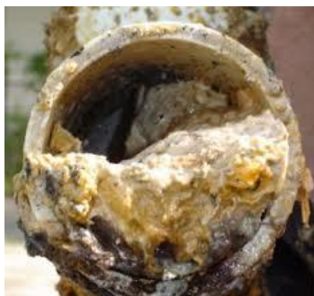
Figure 9: FOG in a sewer
