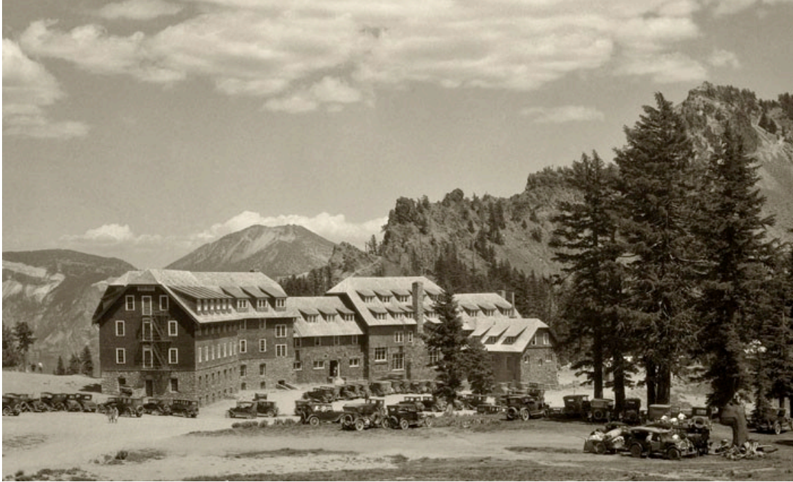
Figure 2.9: Crater Lake Lodge in 1926 showing the 1922 additions to the right. Photograph by Ralph Eddy.
