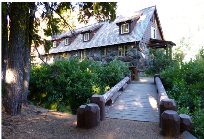
Figure 2.14: Original Ranger's Dormitory (1932), now the Steel Visitor Center. August 2013.
