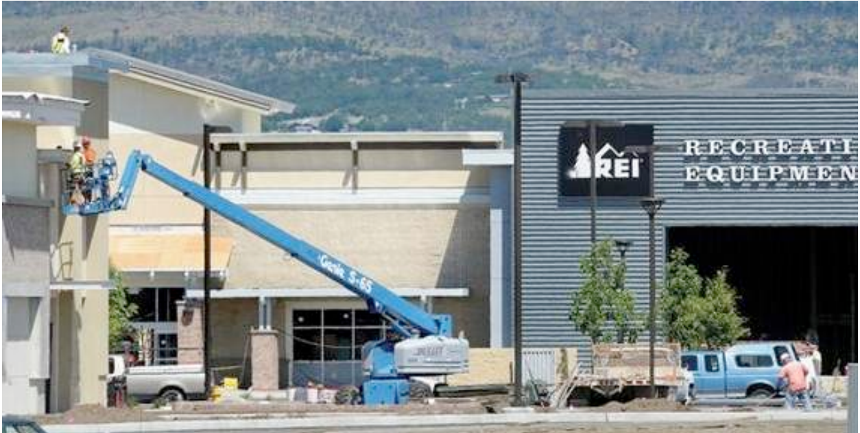
Figure 15: New mall under construction in west Medford, anchored by REI and Trader Joes.
