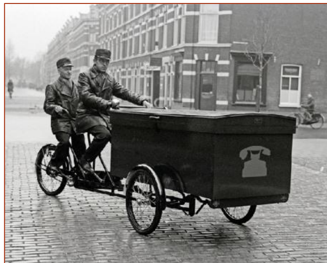
Image 7: Telephone repair unit
