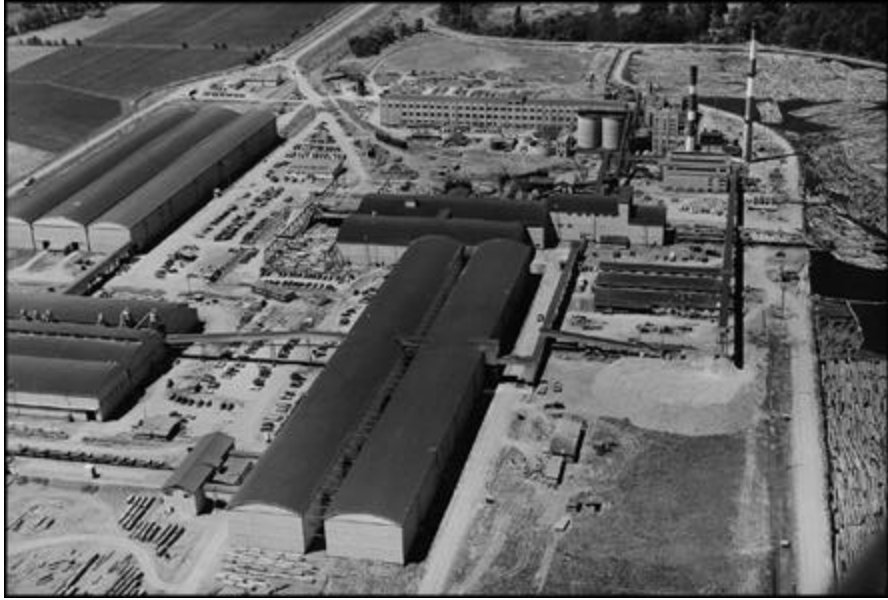
Figure 20. Weyerhaeuser mill facility. (Photo courtesy of the Springfield Museum)
