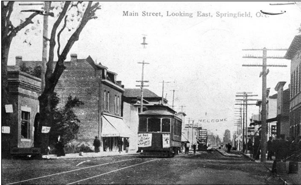
Figure 5. Electric streetcar in downtown Springfield, c.1910. (Photo courtesy of the Springfield Museum)
