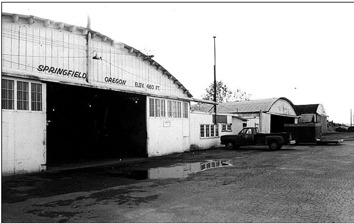
Figure 26. Springfield’s airport, constructed in 1946. (Photo courtesy of the Springfield Museum)
