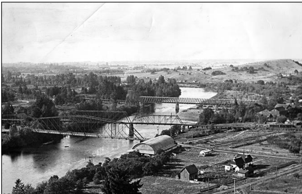
Figure 6. Bridges over Willamette River: wagon road bridge (foreground), railroad bridge (middle), streetcar bridge (background) (Photo courtesy of the Springfield Museum)
