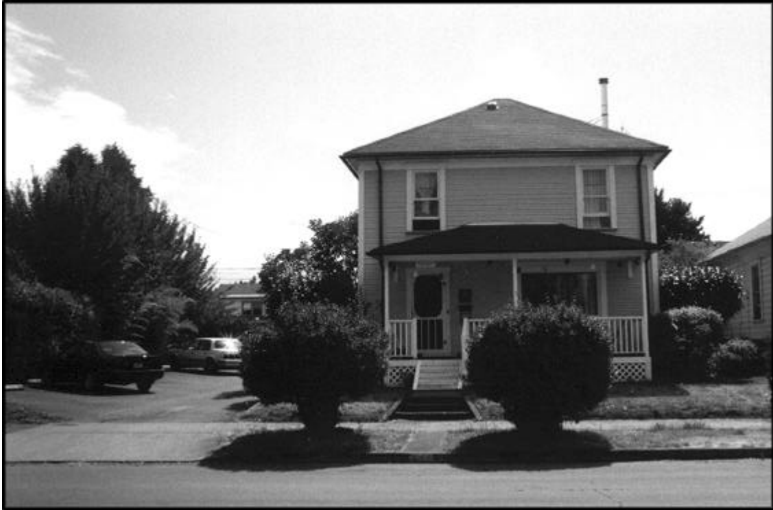
Figure 35. Example of an early American Foursquare style house, located in the Washburne Historic District. (Photo by M. Dennis, 1999)
