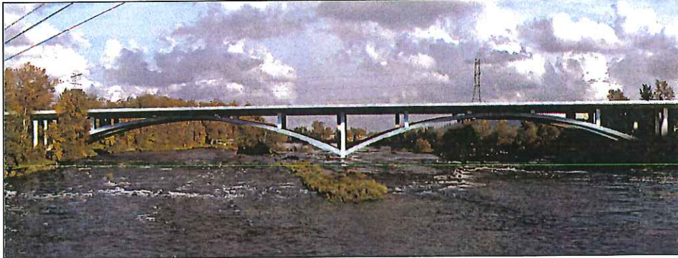
View from Pedestrian Bridge Looking East
