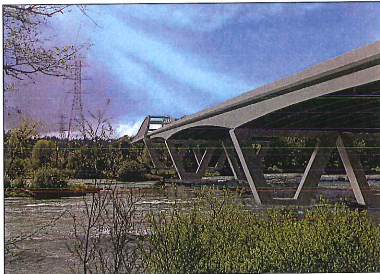
Haunched I Girders Over River View from the Pedestrian Path Looking South
