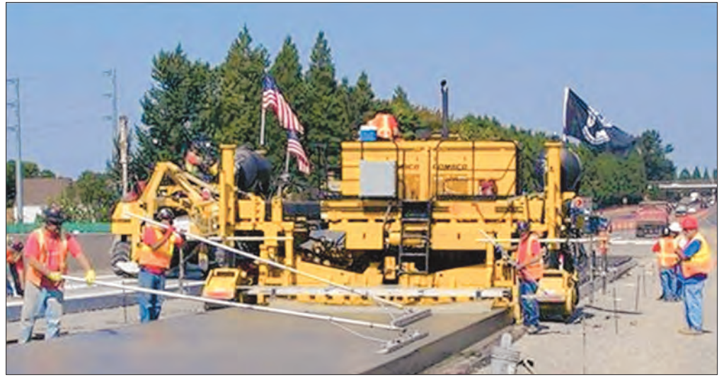
Workers use a large paving machine to create the reinforced concrete roadways leading to and from the bridge.
