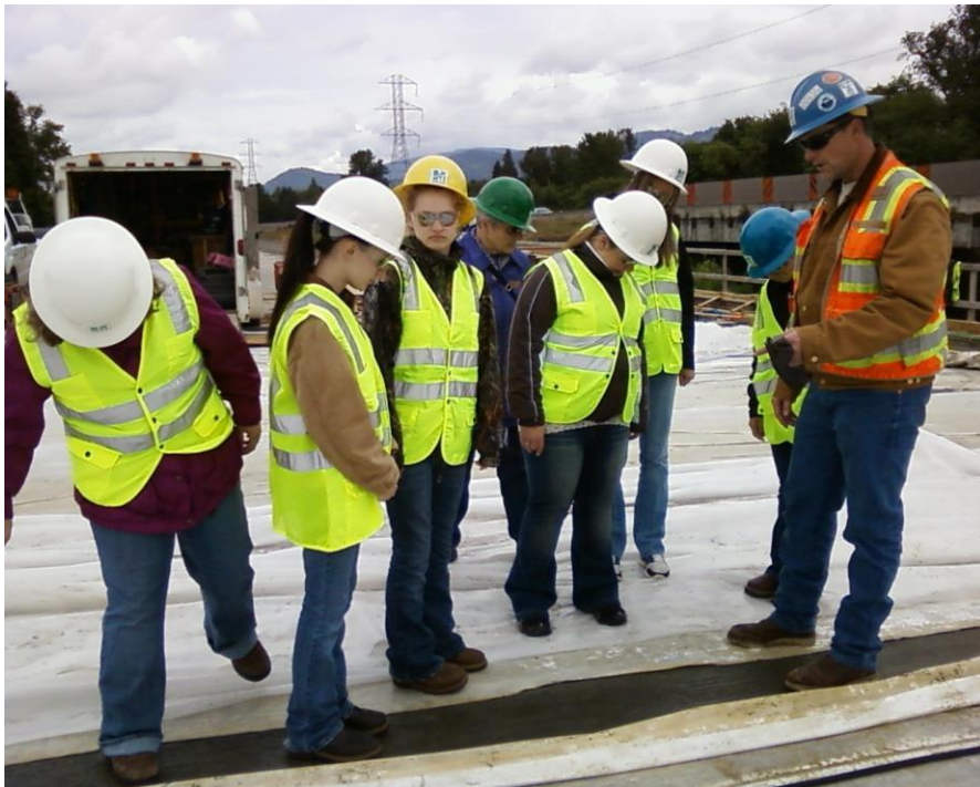
Students get to check out the top surface (concrete deck) of the southbound lanes of the newly built bridge. Note the plastic sheeting to protect recently placed concrete from inclement weather during the curing process
